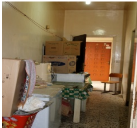
Figure 6.79 Photo shows the clutter in the corridor leading to the entrance
