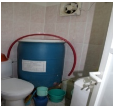
Figure 6.40 Another bathroom with large water storage container
