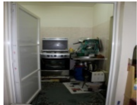
Figure 6.36 Photo shows the kitchen area with piles of utensils covering the gas supply
