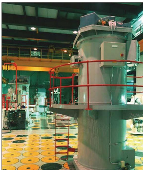
Figure 13: Air-cooled interim storage systems for vitrified HLW at Sellafield (NDA, 2010)
