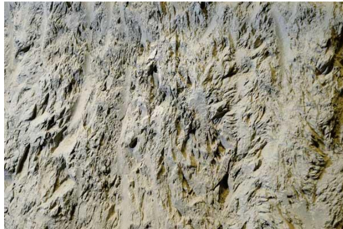
Figure 5: Photo from the Mont Terri Rock Laboratory, open tunnel wall of the Opalinus clay; Picture courtesy of Dieter Enz (Nagra, 2016)
