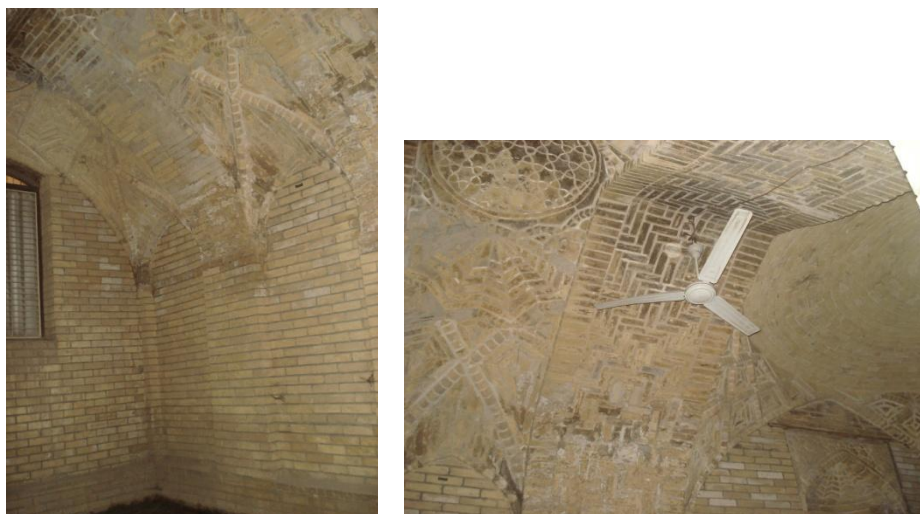
Figure 8.22: Refurbishing the sardab of the T.C.H.T/ Al-Kadhimiya by an Indian company (PH. CH10, 2012), (Author)
