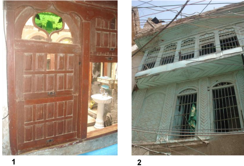
Figure 9.6: Modification and adaptation through alterations caused by way of life in T.C.H.T of the Al-Kadhimiya on moderate days to achieve partial control of the environment by opening the windows for appropriate ventilation, (Author). (1) (PH.CH4, 2012) (2) (PH.CH7, 2012)
