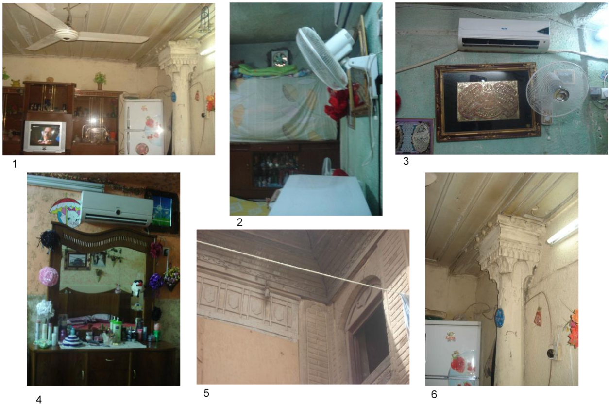
Figure 7.17: Example of refurbishing and types of device in the T.C.H.T in Al-Kadhimiya, House NO. 7 (PH. CH7, 2012), (Author).
