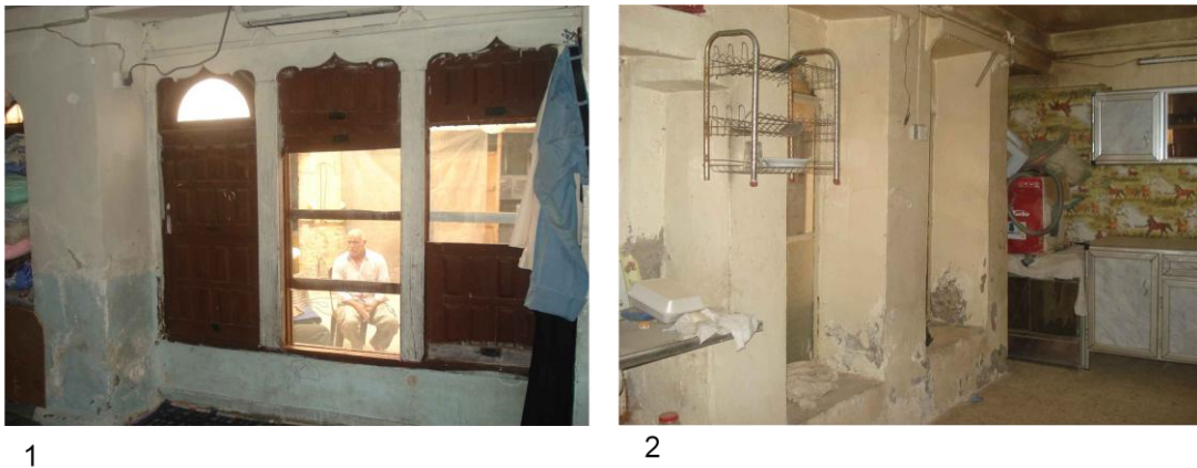
Figure 9.10: Increased the humidity in the ground level leads to environmental challenge for living in T.C.H.T in the Al-Kadhimiya, (Author). (1) Living room (PH.CH.1, 2012), (2) Kitchen (PH.CH.8, 2012)
