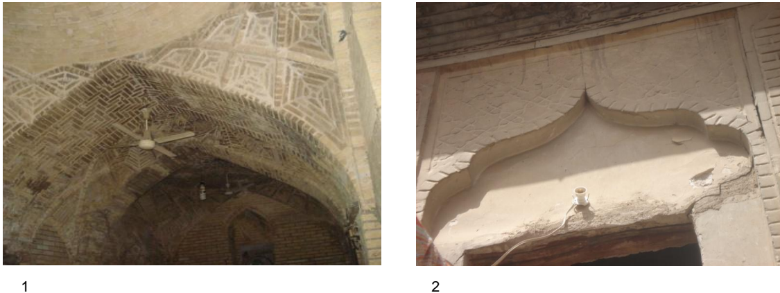
Figure 3.11 Brick ornaments in walls and ceilings in a T.C.H.T. in Baghdad/ Al-Kadhimiya, (Author). (1) (PH, CH.9, 2012) (2) (PH, CH.2, 2012).
