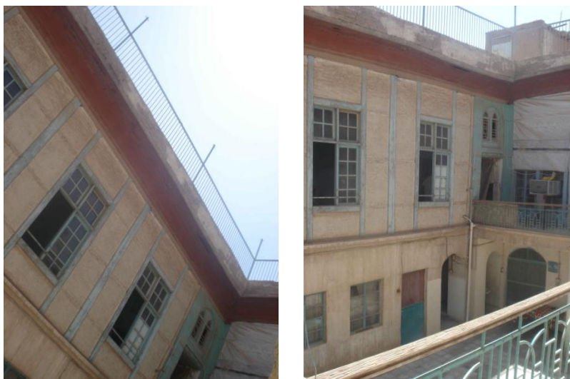
Figure8.12: The size of the courtyard slot in the T.C.H.T in the Al-Kadhimiya making the environmental condition hard to control (PH, CH 8, 2012), (Author).
