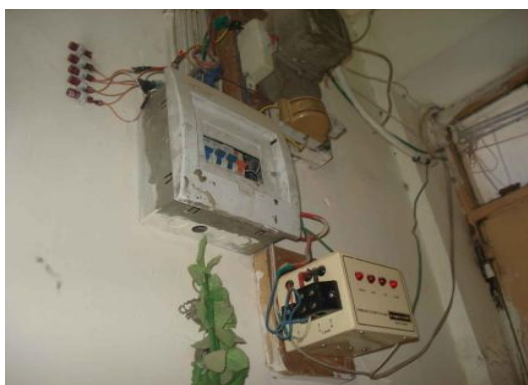
Figure 8.6: Using change over and a stabilizer to provide a stable electricity supply and to avoid power cuts (Ph.Ch.6, 2012), (Author).
