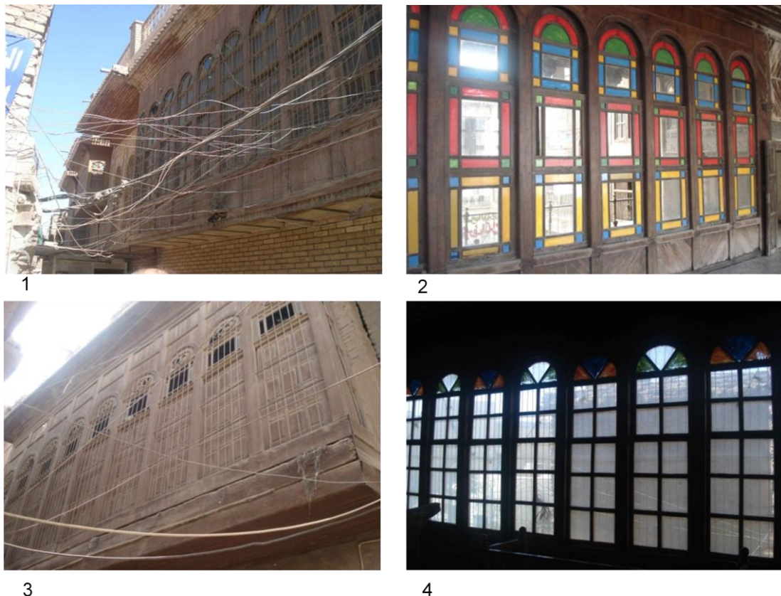
Figure 6.2: The “ Shanasheel ” is an element that response environmentally, socially and aesthetically that is distinctive to the Al-Kadhimiya historical 1+2 (PH.CH10, 2012), 3+4 (PH.CH5, 2012), (Author).
