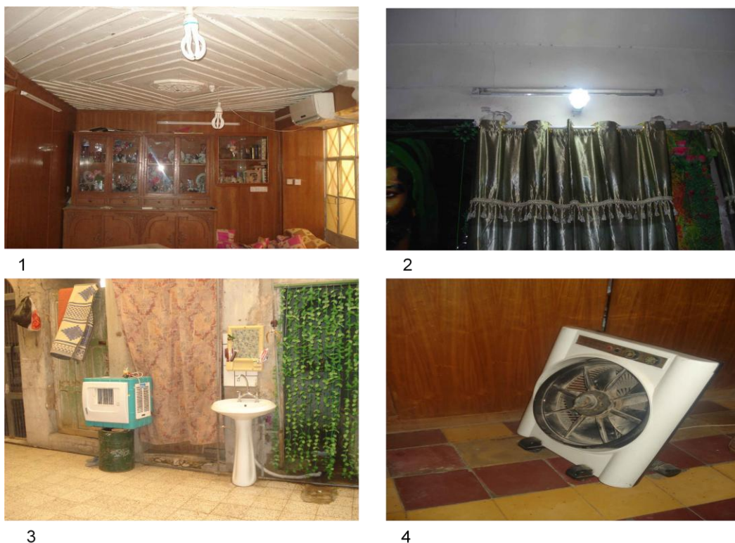
Figure 9.12: An attempt to reduce the energy consumption in the T.C.H.T in the Al-Kadhimiya, which contributed to the environmental challenge, (Author). (A)Using economical lamps (1) (PH.CH.8, 2012), (2) (PH.CH. 6, 2012). (B) Using economical device (3) (PH.CH.5, 2012), (4) (PH.CH.1, 2012)
