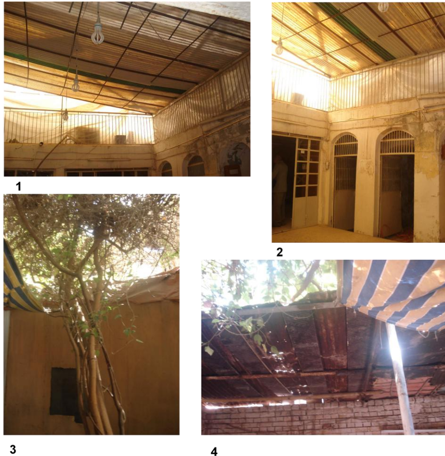
Figure 9.5: Modification and adaptation through alterations caused by way of life in T.C.H.T in the Al-Kadhimiya on harsh weather to achieve partial control of the environment by as a part of lifestyle: Covering the courtyard with nylon sheeting in winter, (Author). (1-2) (PH.CH. 8, 2012) or tent in summer to avoid harsh weather (3-4) (PH.CH. 3, 2012)
