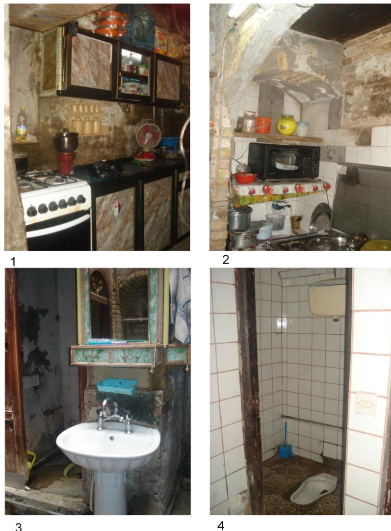
Figure 9.11: Lack of adequate space leads to environmental challenges through the difficulty of controlling the indoor environment quality when living in the T.C.H.T in the Al-Kadhimiya, including increased humidity and odour level, (Author). (A) In kitchens (1.) (PH.CH.5, 2012), (2.)(PH.CH.4, 2012) (B) In the toilet or bathroom (3.) (PH.CH. 4, 2012), (4.) (PH.CH.10, 2012)
