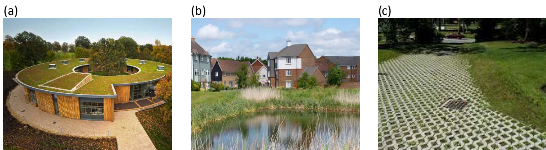
Figure 2-15. Examples of BGIs that can be applied in urban environments: (a) green roofs (source: https://goo.gl/994Sck ); (b) retention basins (source: https://goo.gl/FVaGYW ); (c) permeable pavement (source: https://goo.gl/azp3m5 ).
