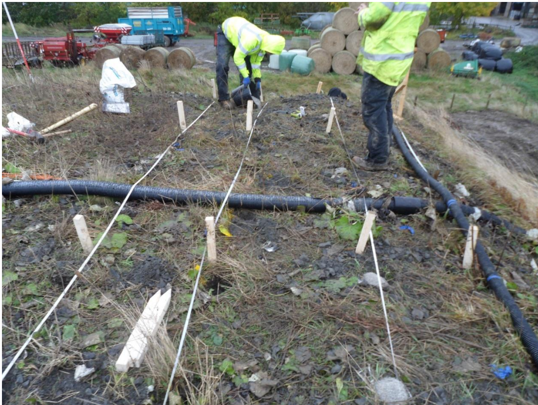
Figure 4.43 ERT electrode installation on crest
