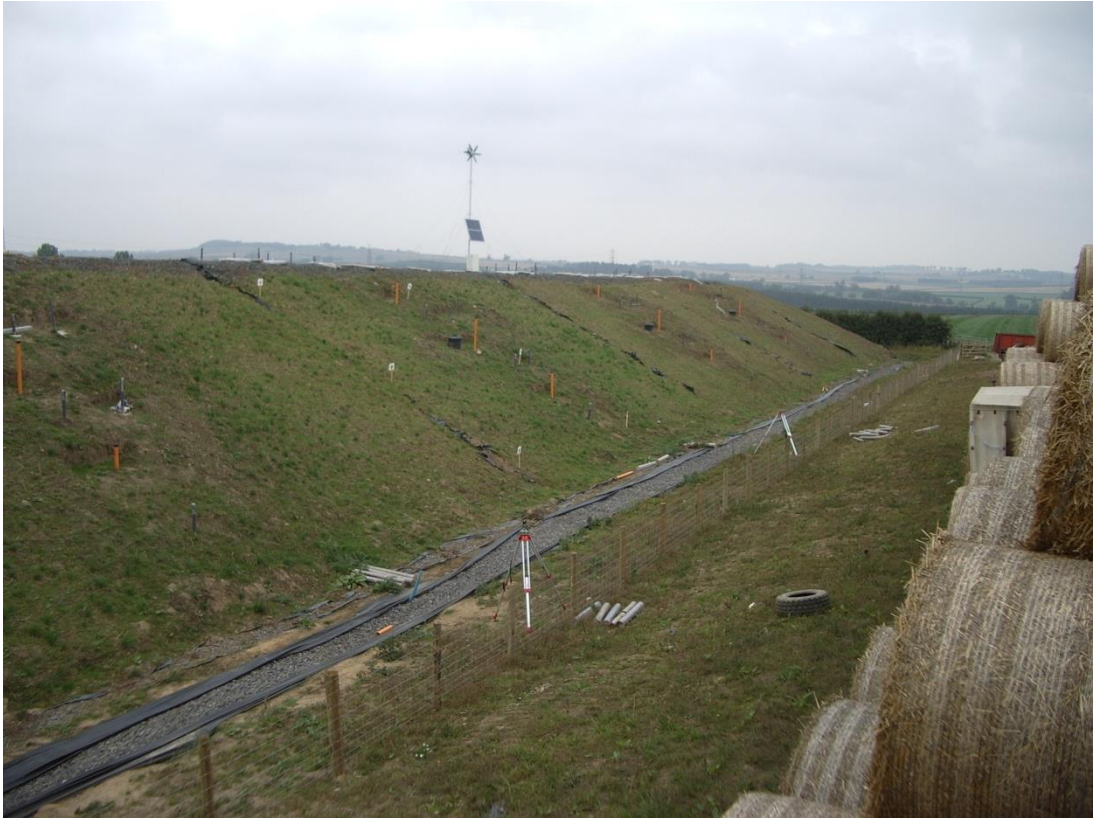
Figure 3.15 Embankment one year after construction (September 2006), showing grass coverage
