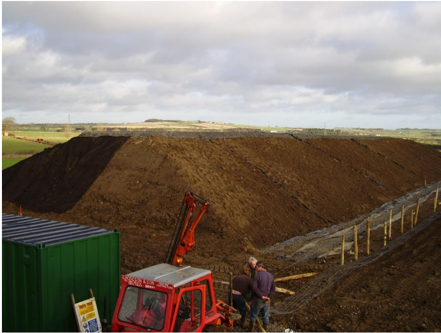
Figure 3.13 Completed embankment, view taken from a point Southwest of Panel A
