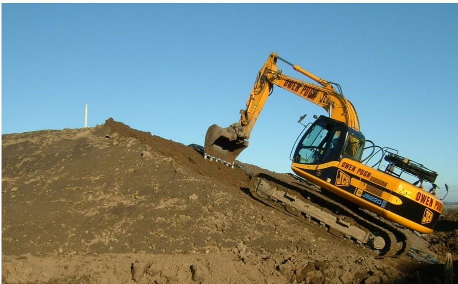
Figure 3.10 Placement of topsoil layer on embankment flanks
