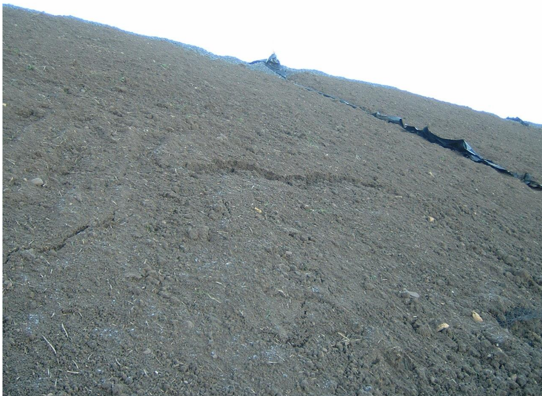
Figure 3.14 Tension cracks in Panel A South flank (November 2005)
