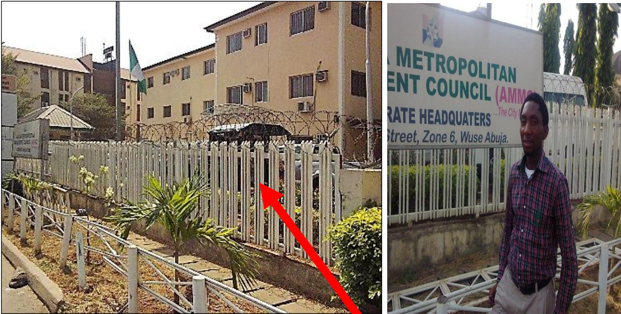
Figure 9: Head Office Department of Development Control, Abuja (DDC); Source: Author, 2013
