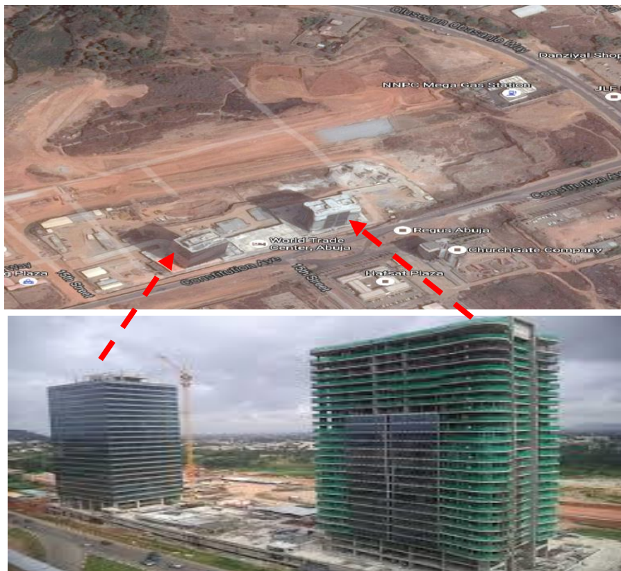
Figure 47: AWTC Mixed development under construction.
