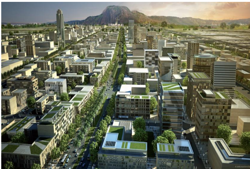
Figure 40: Abuja boulevards (streets lined with trees).
