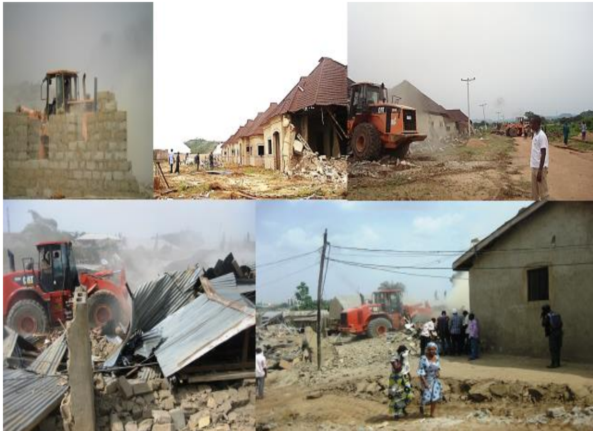
Figure 15: Site oriented nature of the planners; planners out for demolitions; Author, 2014
