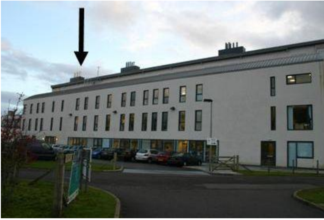
OBAN antenna installation which is approximately 15m above ground level.
