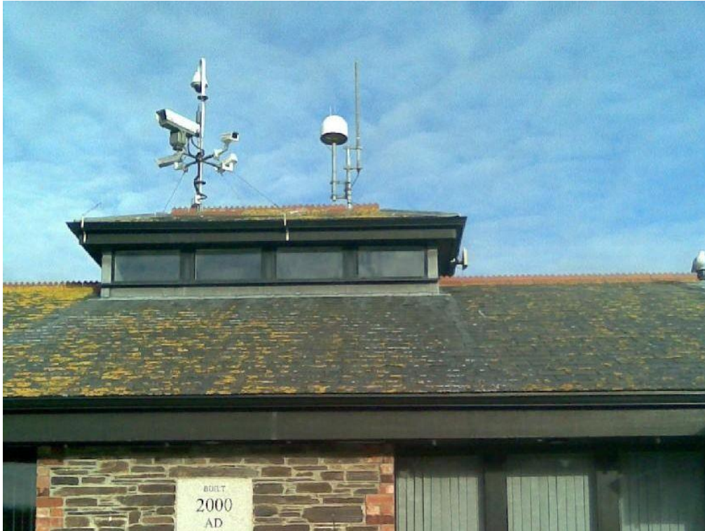
PADT antenna installation which is approximately 5m above ground level.
