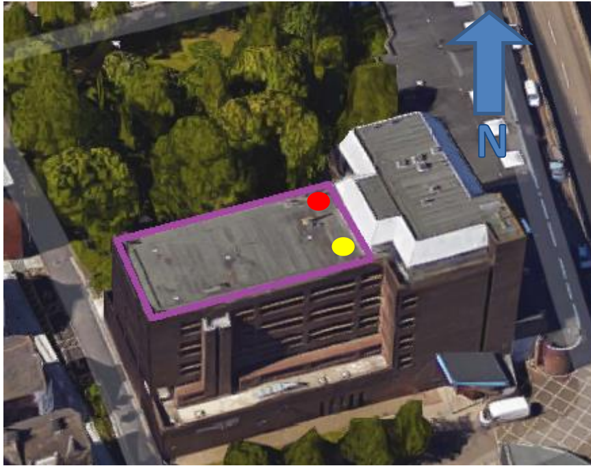
Figure 5.1: Aerial photograph of the Drummond building's flat roof, outlined in purple. The North East antenna location (DRMS) is in red and the South East antenna location (DRMB) in yellow. Copyright Google.
