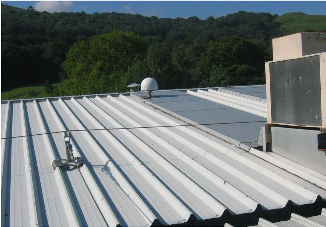
MACY antenna installation which is approximately 12m above ground level.
