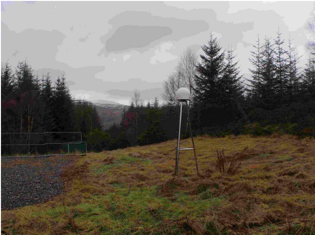
KILN antenna installation which is approximately 2m above ground level.
