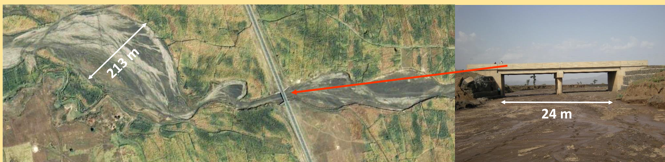
Fig. 8 Gereb Oda R. and road bridge in 2008
