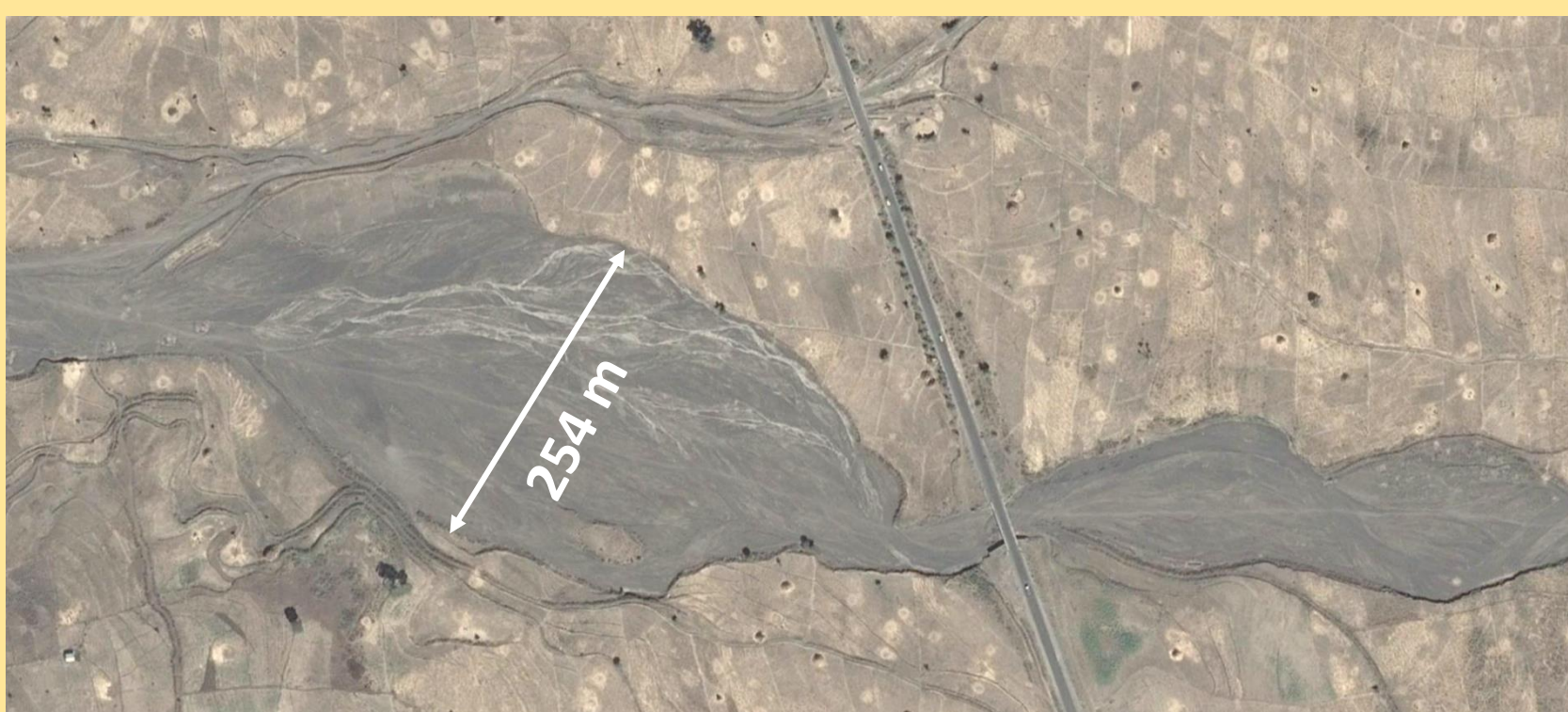
Fig. 9 Gereb Oda R. and road bridge in 2015
