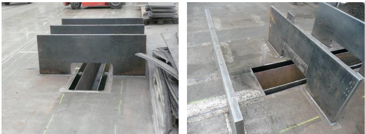
Fig. 6. Removal of cracked parts of deck plate
