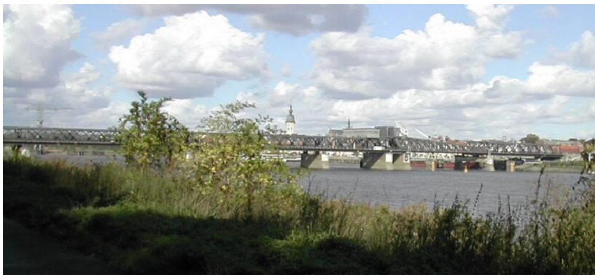
Fig. 2. Overview of truss bridge built 1955
