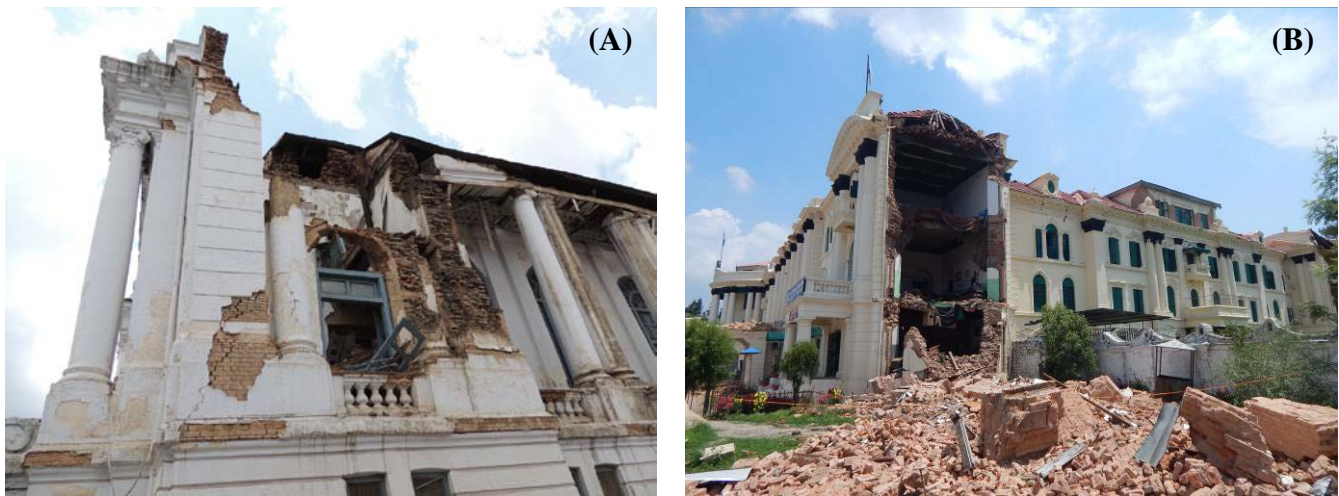
Fig. 11: (A) Extensively damaged Hanuman Dhoka; (B) Out-of-plane collapse in Nepal Academy of Fine Arts
