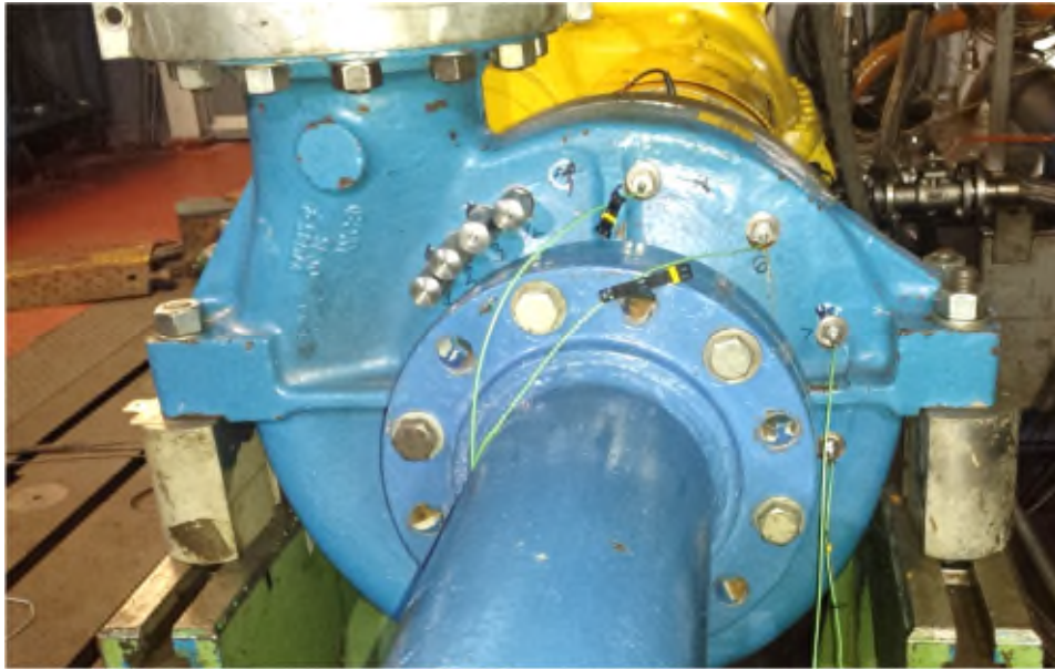
Figure 31 Photograph of the pump set up with pressure transduces in positions C5- C8
