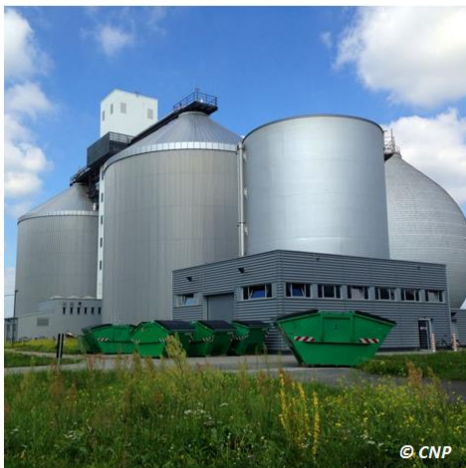
WWTP Berlin Wassmansdorf
