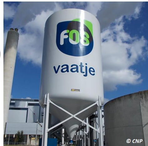
WWTP Amsterdam West
