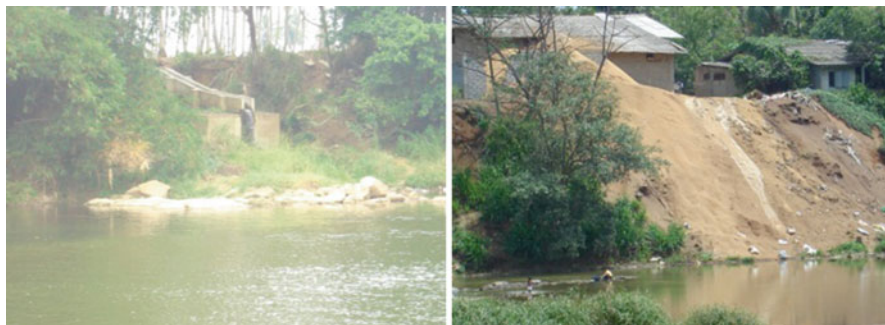
Fig. 9.6 Industrial waste discharge
