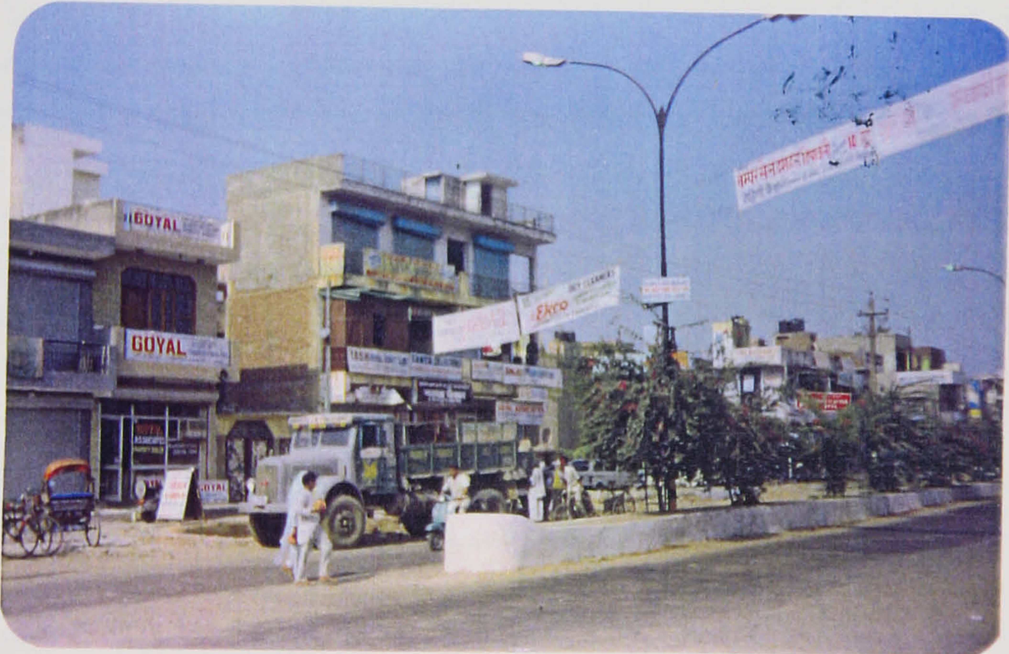
Picture above shows residential space misused violating both use criteria and permitted floors along major access roads at Rohini, Delhi
