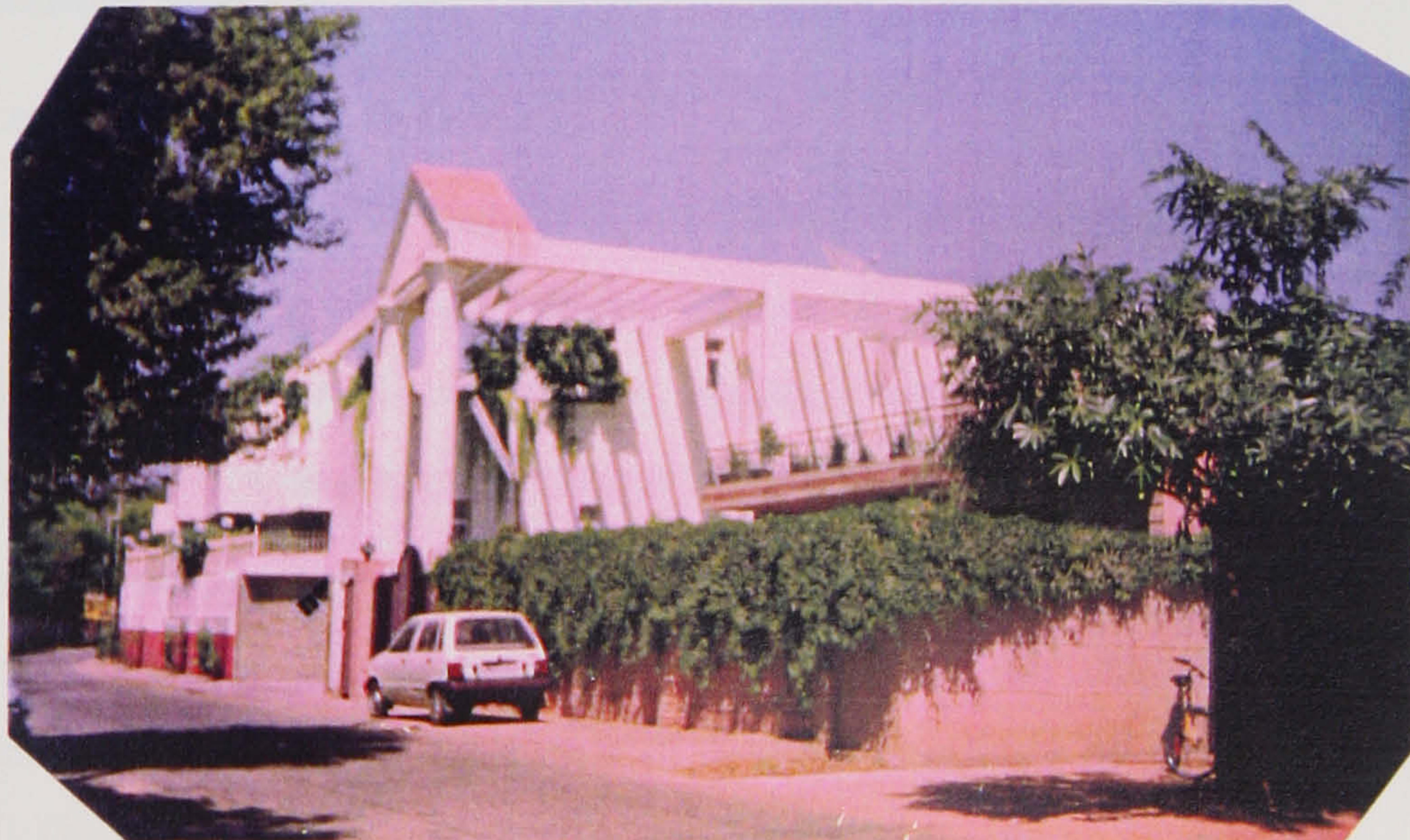
Picture above shows high standard unauthorised developments at Sainik Farm, South Delhi
