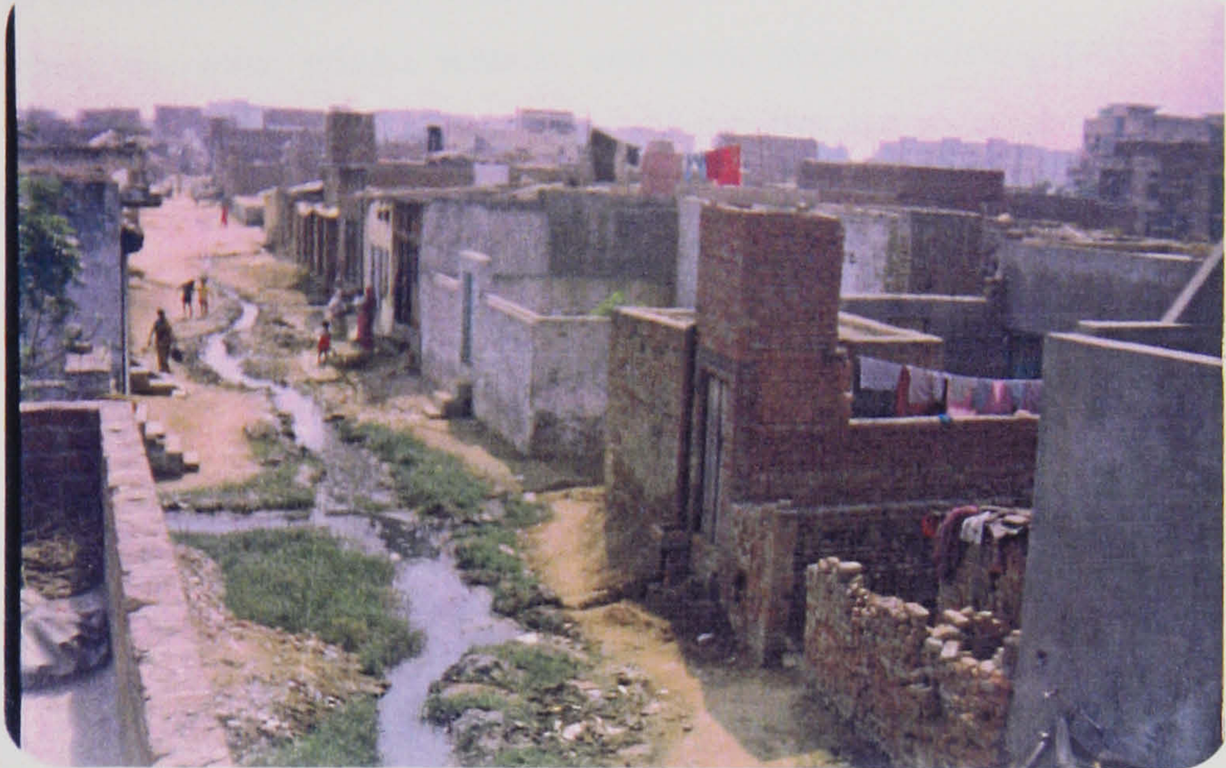
Picture above shows poor condition of drainage and water logging in a new unauthorised colony
