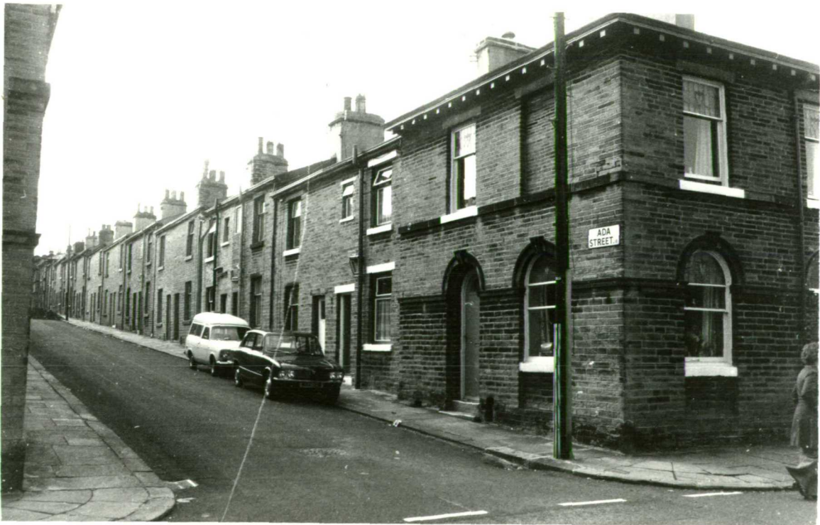
Figure 73 2 bedroom houses in Ada Street.
