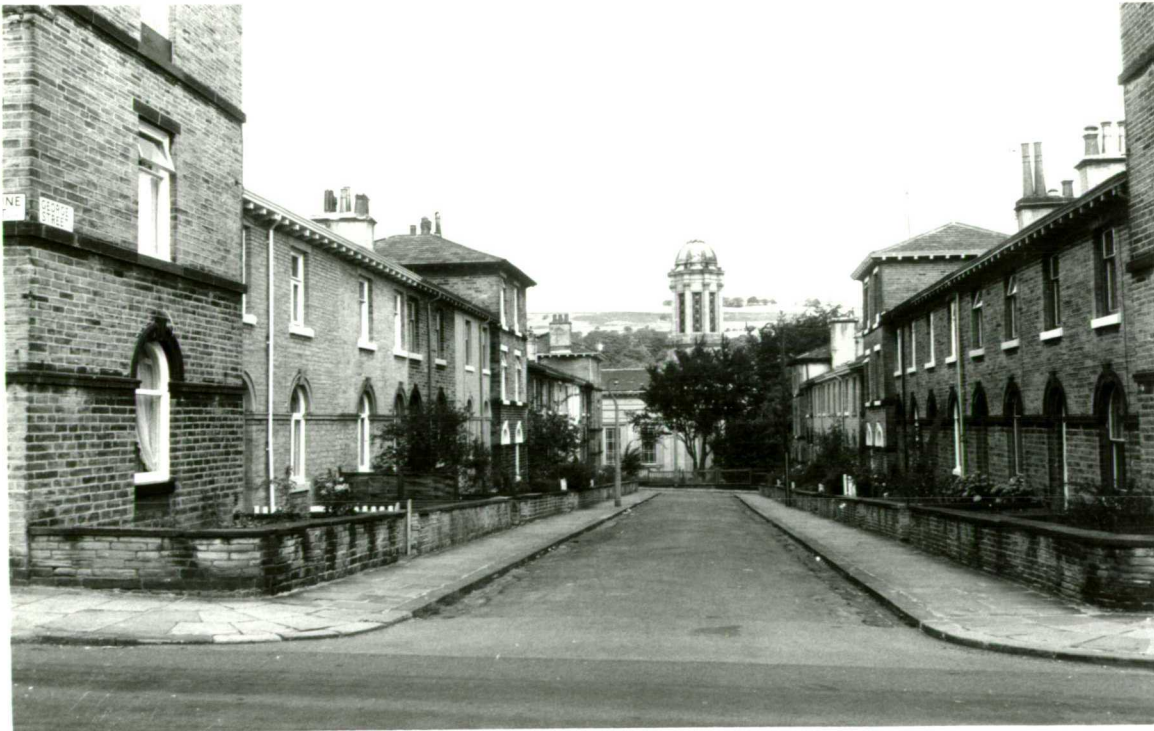
Figure 70 View along George Street of Saltaire Congregational Church.
