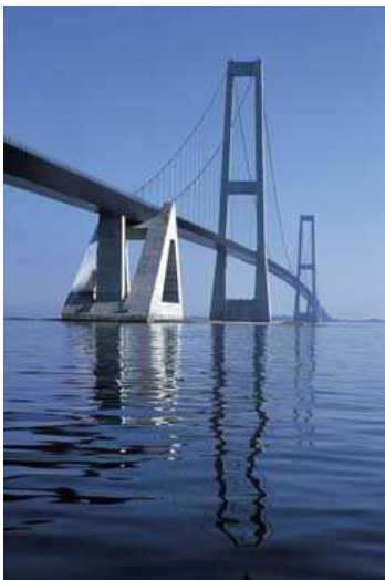
Fig. 1: The Great Belt Bridge (Denmark)
