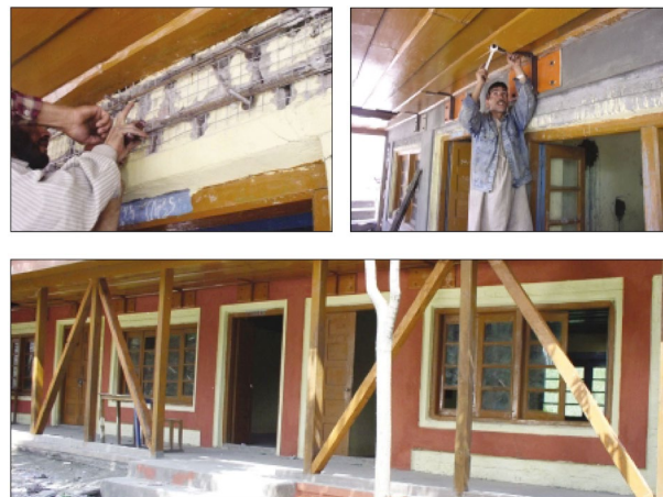
Figure 7. Strengthening with belts, roof anchoring and diagonal timber bracing [7]
