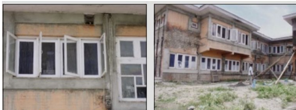
Figure 8. Strengthening with belt encasement around openings [7]
