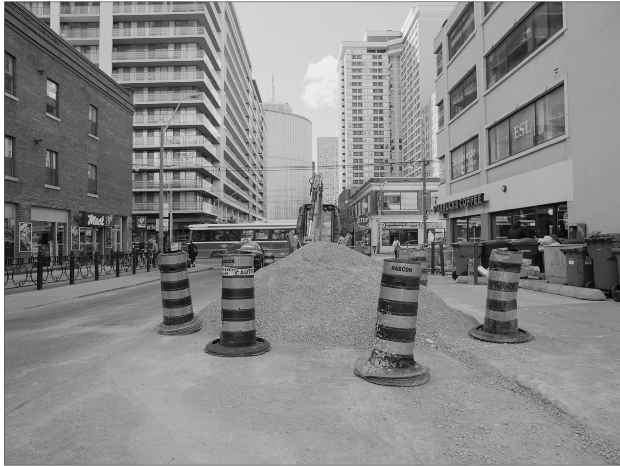
FIG 5 Elizabeth Street North of Dundas Street and New City Hall, 2011
