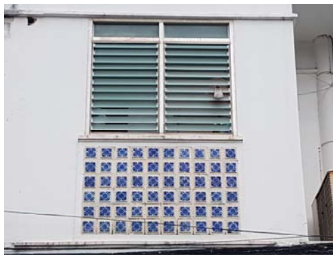
Figure 4. Typical example of louvre windows used for housing developments in urban areas of Thailand.
