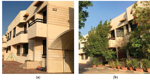
Figure 1. Plant-shaded façade in comparison with unshaded façade of identical housing units, Al-Ain, where (a) Unshaded building façade (bare wall), (b) Plant-shaded façade (plant-shaded wall).
