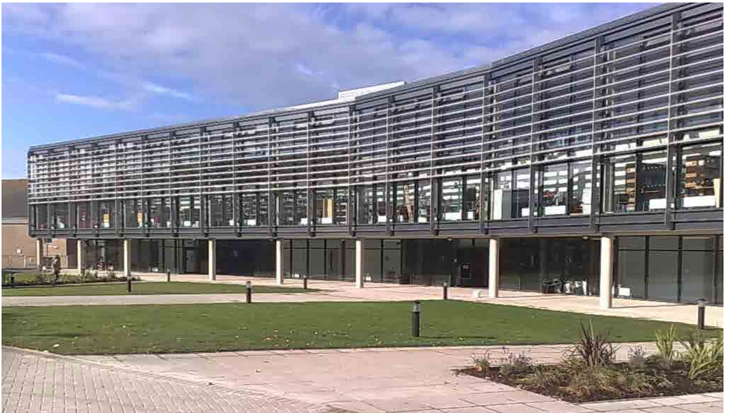
The Checkland Building at Falmer campus, University of Brighton
