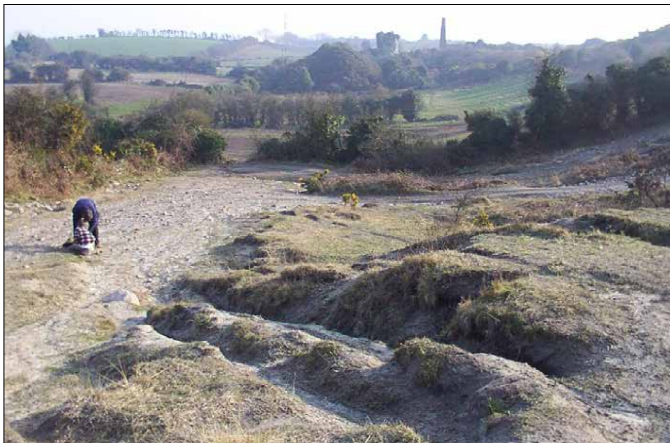
Fig. 3: Eroded tailings impoundment in the area southeast of the South Engine Shaft chimney stack, looking south with the Bog Shaft engine house, chimney stack and (gorse-covered) spoil heap visible in the distance. During periods of rain, cerussite-rich tailings material is washed downslope through the gap in the hedge into the 'meadow' beyond. The meadow and hedge are the subjects of biogeochemical analyses reported here
