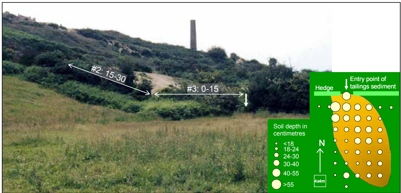
Fig.8: Photograph taken in 2000 of the meadow looking northwest with the prominent South Engine Shaft chimney stack on the escarpment. Central in the photograph, the pale area bare of vegetation is an eroded tailings impoundment. Extending left to right is the hedgerow through which eroded tailings are washed into the meadow. Vigorous growth of pale green bracken is visible in an area where sandy, calcite-rich tailings have been deposited. Arrowed lines labelled 0-15 and 15-30 indicate lengths of hedge from which vegetation samples were taken for analysis (Fig. 11). Inset: map of the redeposited tailings plume in the meadow showing soil depths estimated by probing on a 4 m grid with an iron rod. The south-eastern extremity of the plume corresponds to the location of the photographer
