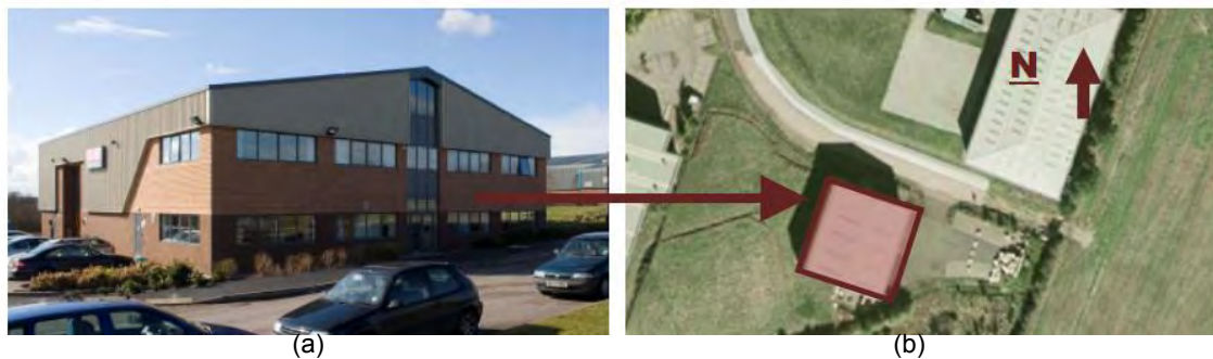
Figure 1: Case study building
