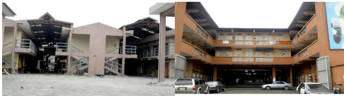
Figure 4. A Section of Remodelled Market South and North Respectively.
