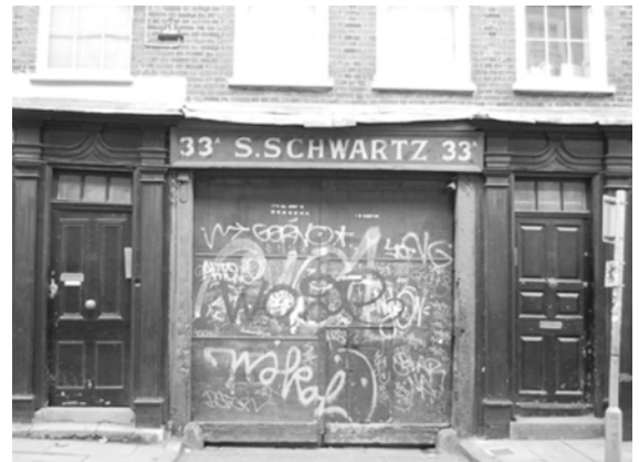
Photograph depicting a shop façade on Fournier Street still retaining the original fascia sign from the Jewish occupation, now covered in graffiti.
