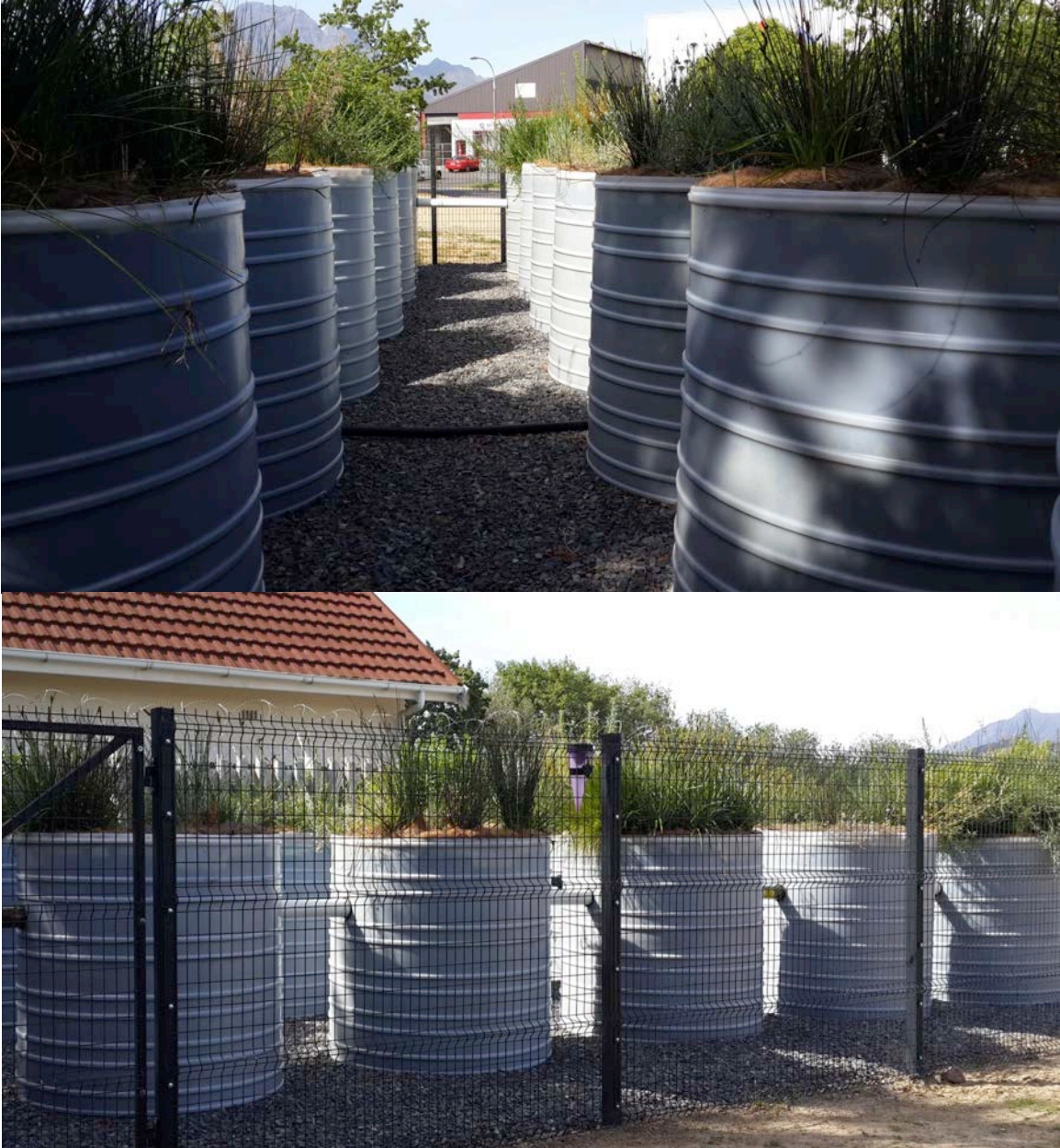
Figure 4: An Eco-Machine matrix at the Plankenberg pilot site. Eerste River water is pumped through the system connected by pipes.
