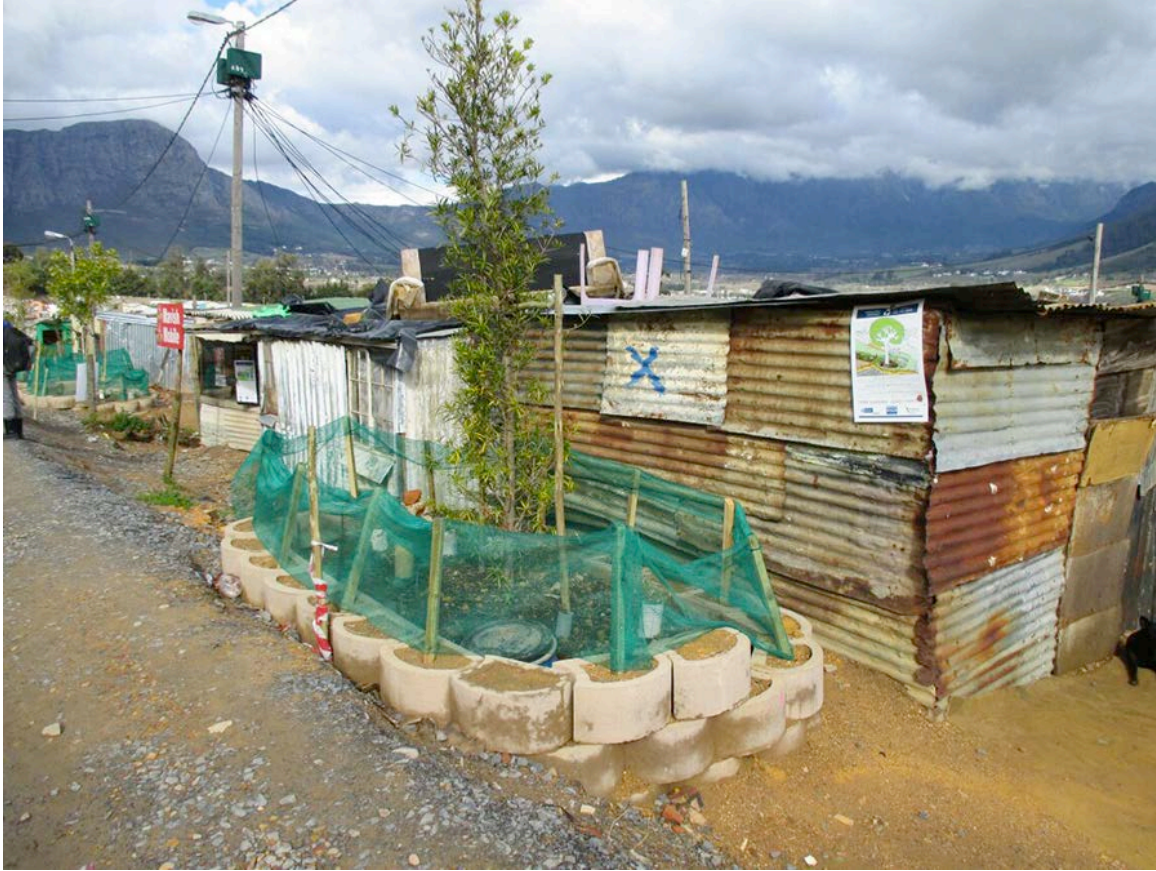
Figure 5: An example of a “tree garden”. Underground pipes fed by ad hoc sewers pass through these systems. The purpose of the gardens is to provide initial greywater treatment and provide green space ( http://www.acturban.com/genius-of-space-berg-river/ , accessed 1/10/2016).
