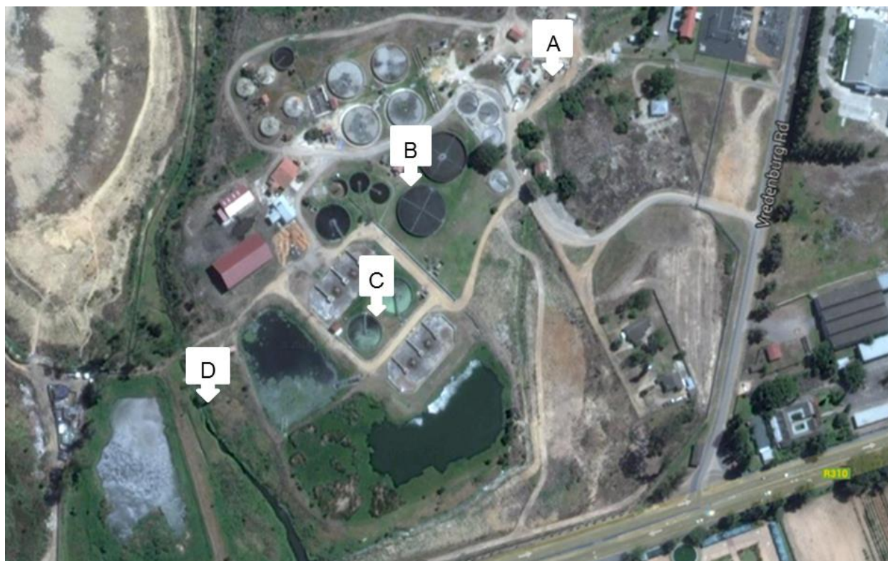
Fig. 2.1. Stellenbosch wastewater treatment plant with sampled sites indicated by A: Influent point; B: Biological trickling filter; C: Aeration tank; D: Effluent point (GPS co-ordinates - 33.943505, 18.824584)
