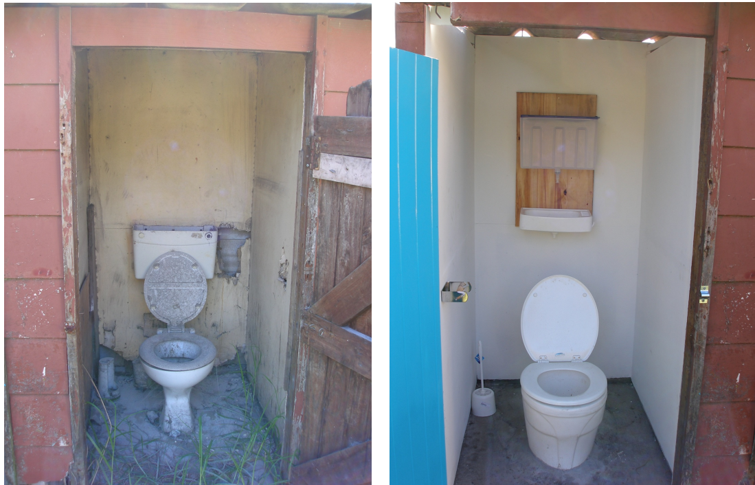
Photos 4.14 and 4.15: Community facilities before and after installation of biodigester (Site B)
