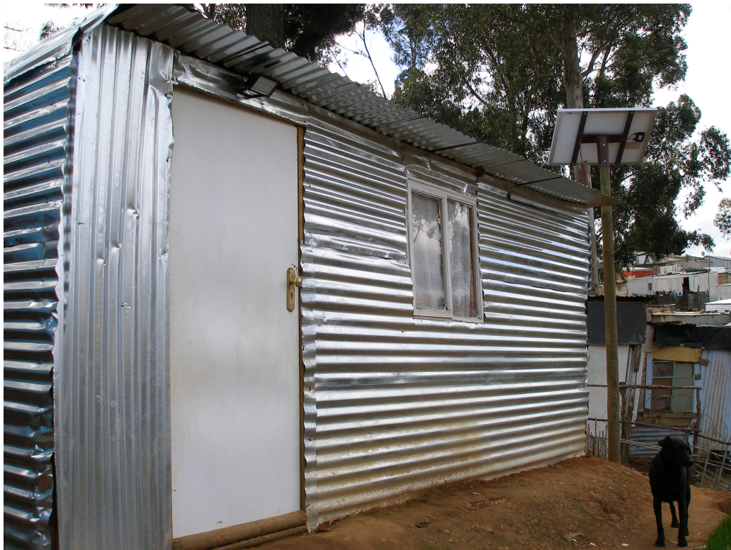
Photo 4.13: External view of iShack incorporating solar energy (Site A)
