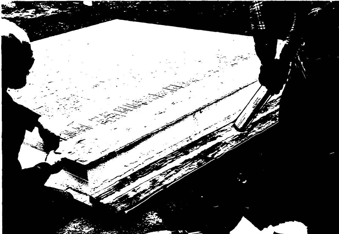
Figure 4-13 Sealant Installation
