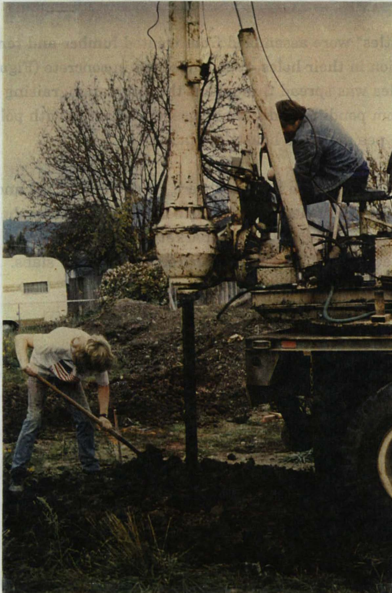
Figure 4-2 Foundation Pier Drilling
