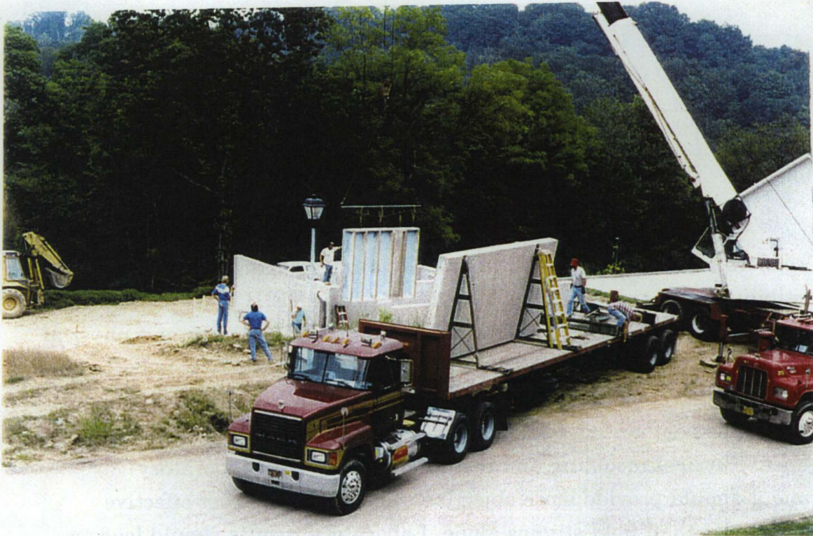
Figure 6-6, Superior Wall Insulated Concrete Foundation
