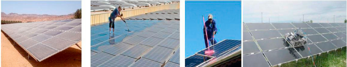
Fig. 2. (a) Dust on PV; (b) brush cleaning; (c) cleaning in BAPV; (d) robotic cleaning in open rack PV.
