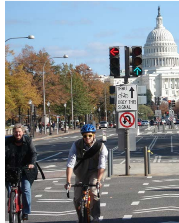
Buffered bike lane on Pennsylvania Avenue in Washington, DC connecting the White House and the US Capitol. Photo: Ralph Buehler.
