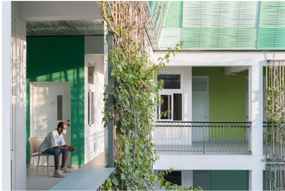
Figure 49 : Gheskio TB hospital ventilated walkways
