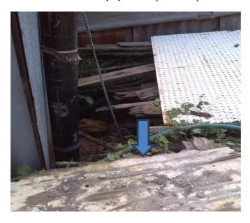
b) Ingress of soil into the VIP pit, i.e. soil particles are visible in the VIP pit – point to the compromised side walls of the toilet facility and possible collapse.
