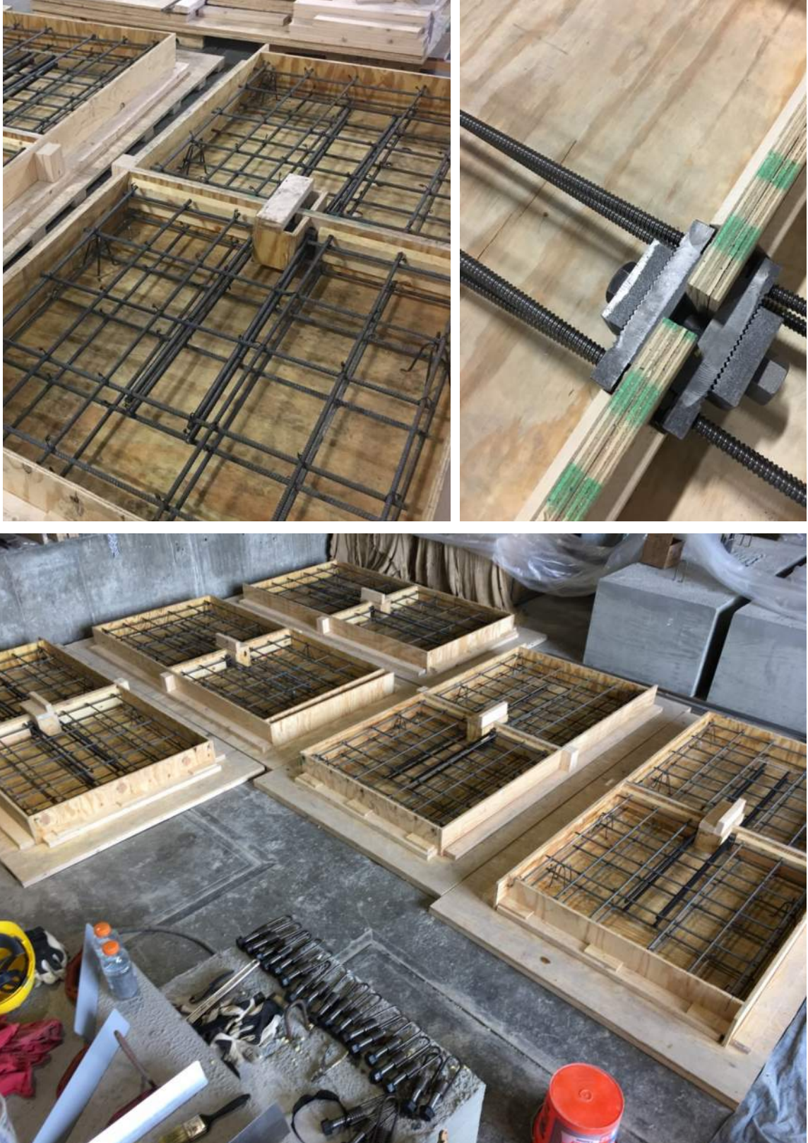
Figure 3.5: Formwork for Mechanical Connection Slab Panels
