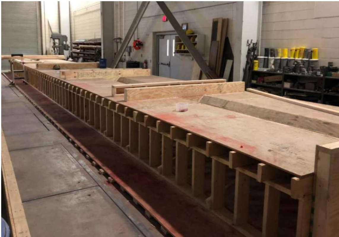
Figure 4.3: Full-Scale Formwork Assembly
