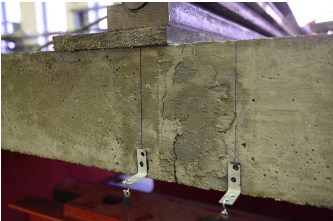
Figure 3.31: Initial Cracking at the Grout Interface (Specimen C-C-2)
