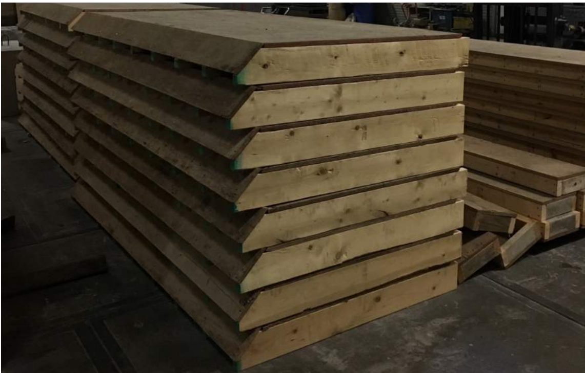
Figure 4.2: Formworks for Full-Scale Bridge Specimens
