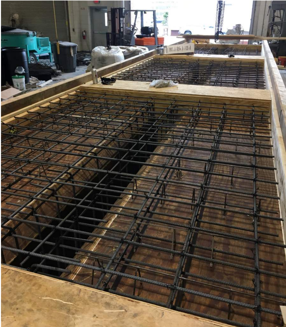
Figure 4.5: Steel Reinforcement Assembly Placed in Formwork
