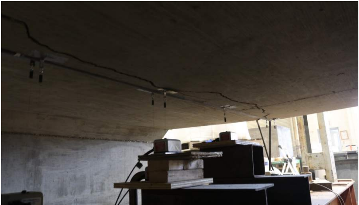
Figure 4.16: Close-up view of the Grouted Joint (Specimen F-M)
