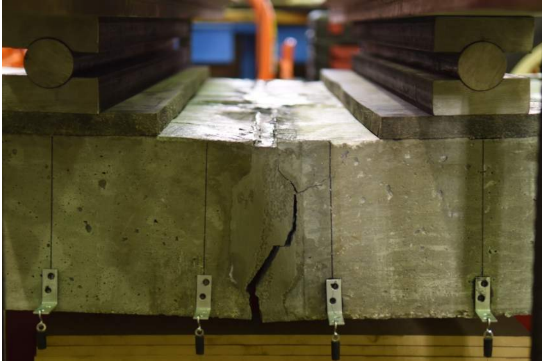
Figure 3.20: Crack Propagation through the Grout (Specimen C-C-1)
