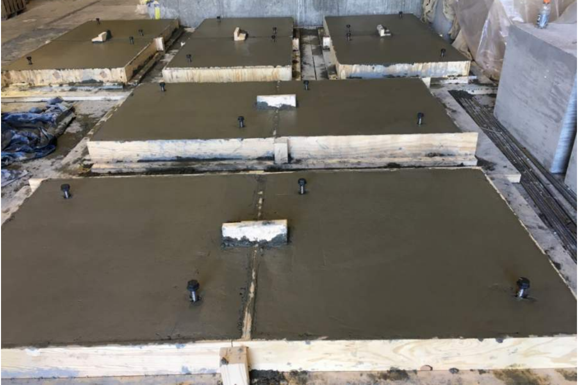
Figure 3.6: Finished Slabs After Anchor Placement
