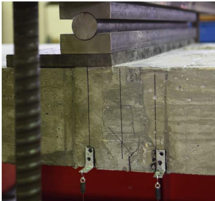
Figure 3.37: Inclined Cracking through the Grout (Specimen F-F-2)
