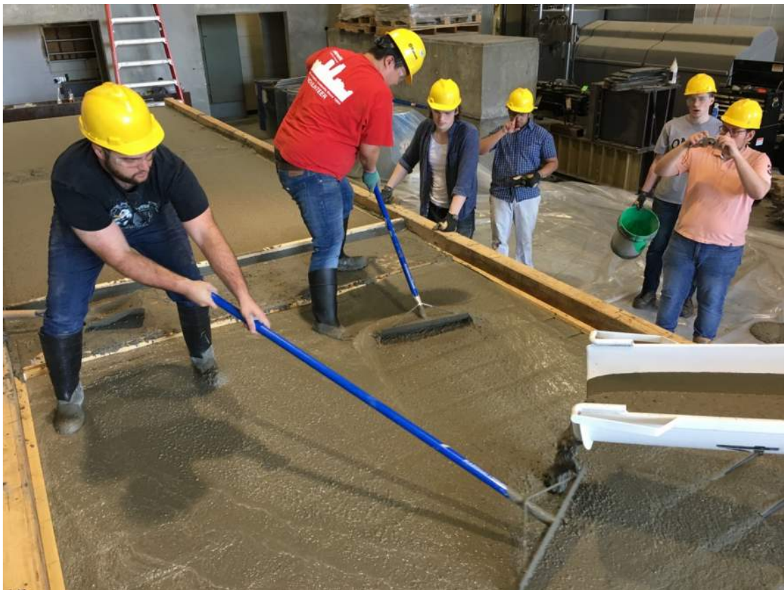
Figure 4.7: Casting Self-Consolidating Concrete for Full-Scale Bridge Specimens
