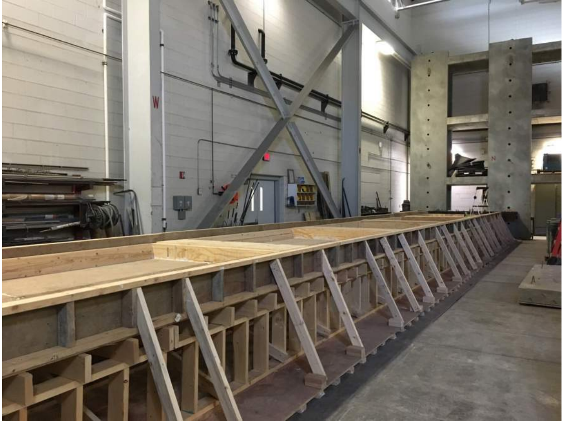
Figure 4.4: Complete Full-Scale Formwork for County Bridge Specimen
