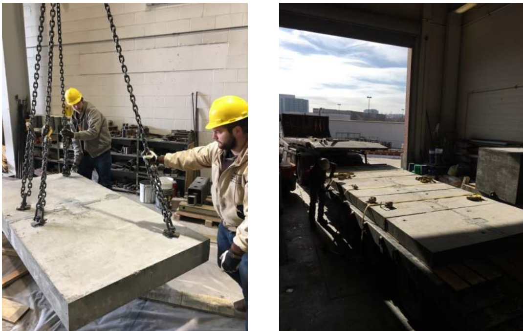
Figure 3.8: Slab Transportation
