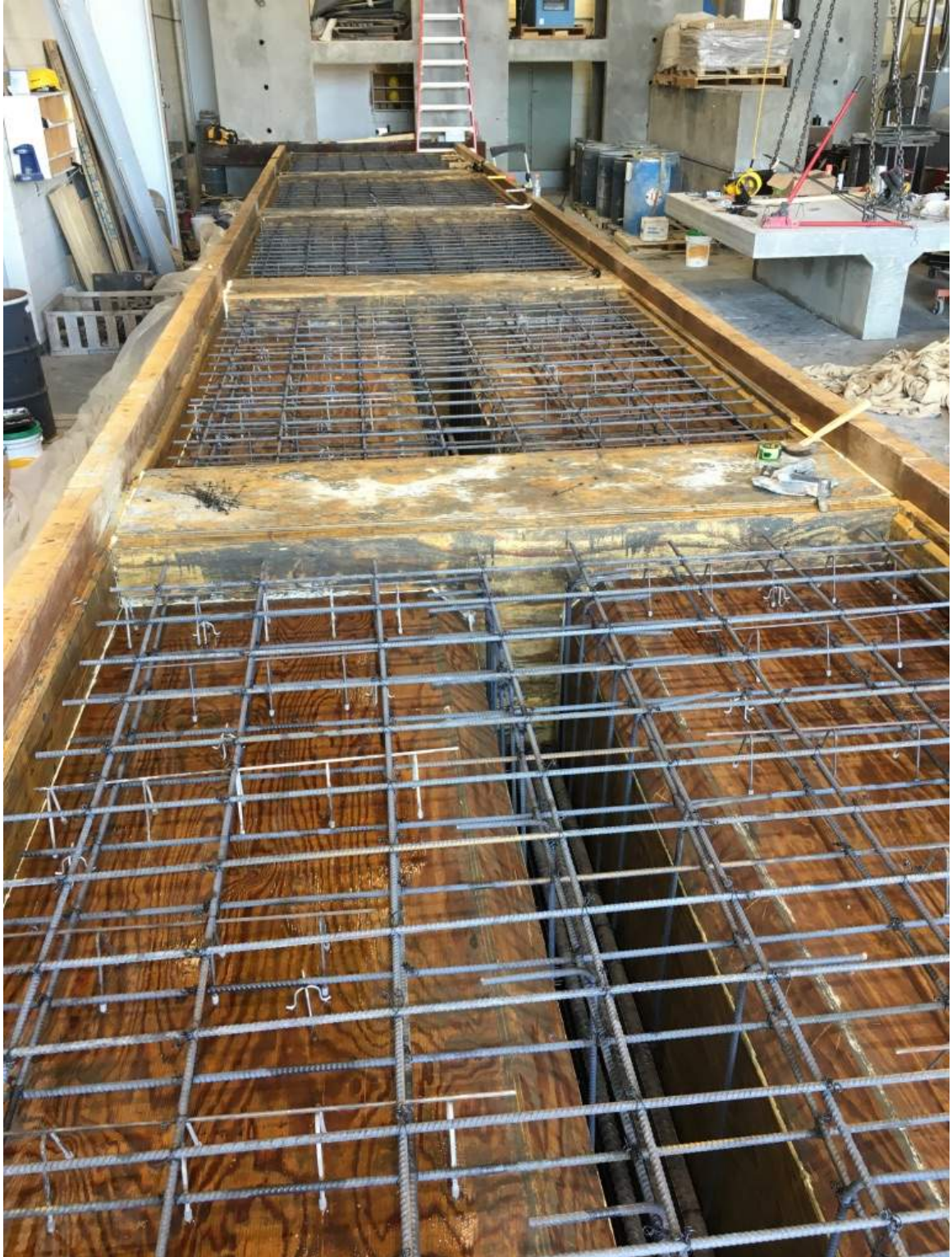
Figure 4.9: Steel Assembly for the Second Pour
