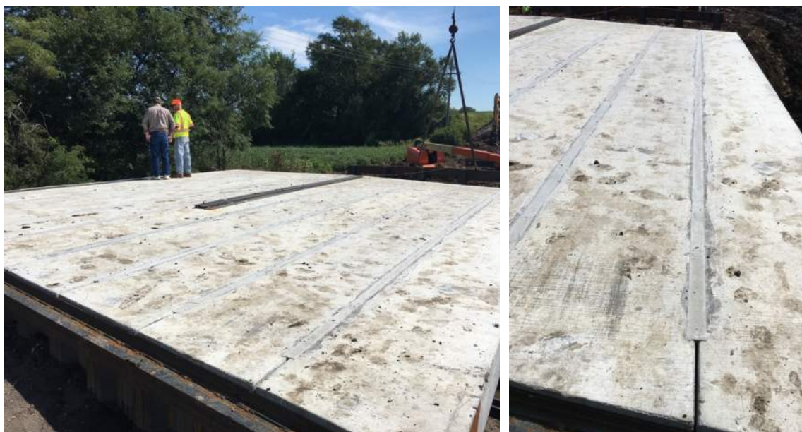
Figure 1.3: Grouts between Longitudinal Shear Keys
