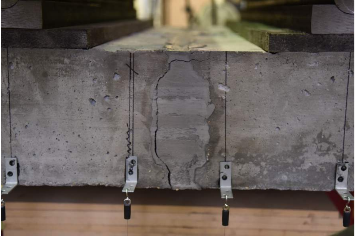
Figure 3.26: Initial Cracking at the Grout Interface (Specimen C-F-1)
