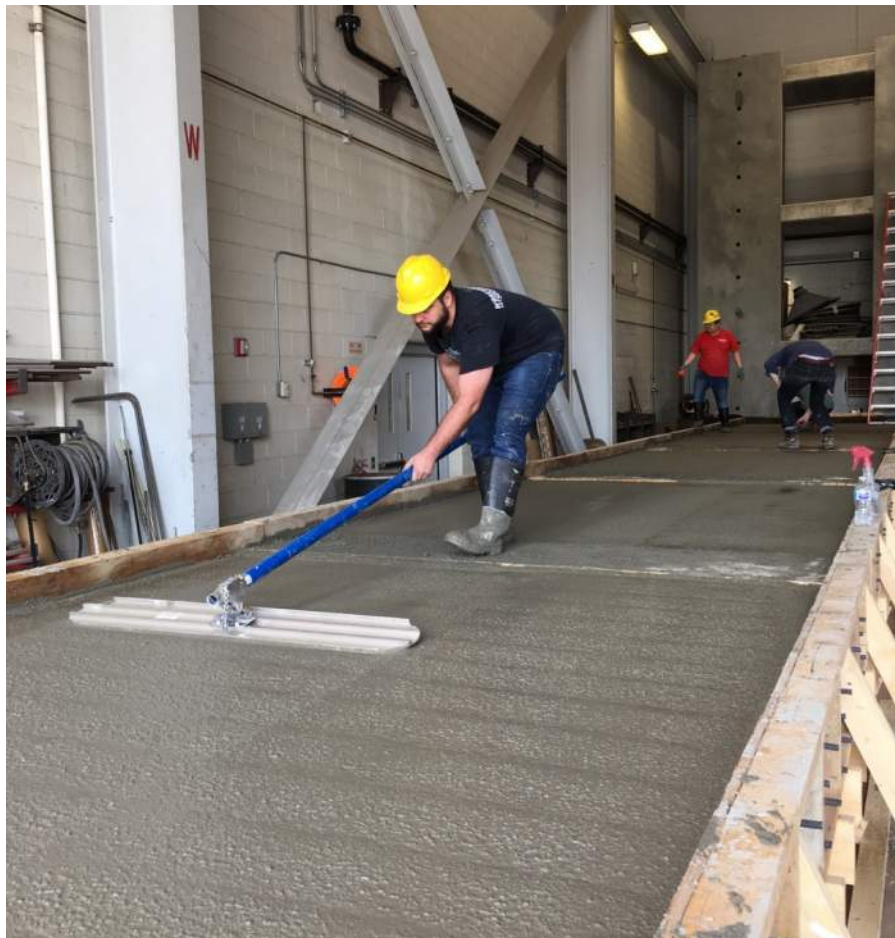
Figure 4.8: Finishing the Full-Scale Bridge Specimens
