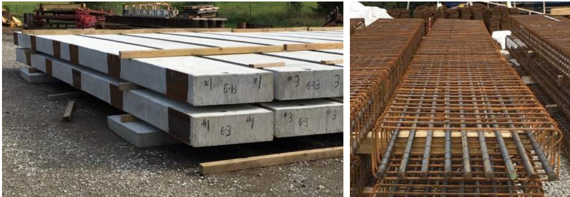
(a) Planks used in multi-beam bridges in Nebraska
