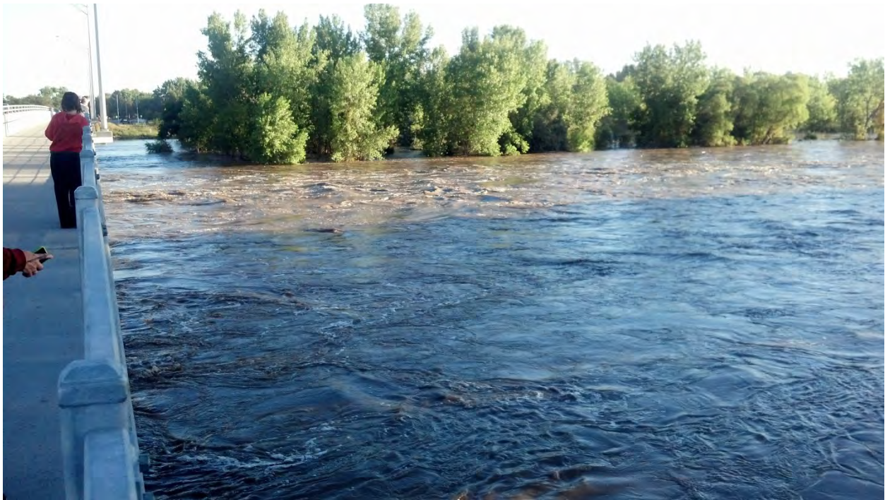
South Platte River Bridge at Buffalo Bill Road, North Platte. September 21, 2013, 9am. Photo courtesy of Kent Miller, Twin Platte NRD.
