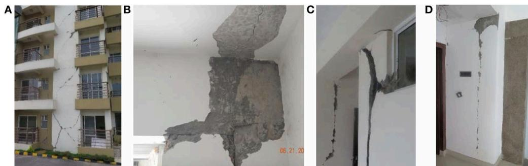
**FIGURE 2 | Observed damage on different components of the building. (A)** Exterior damage. **(B)** Beam-column joint. **(C)** Interior infill wall. **(D)** Separation between column and infill.
