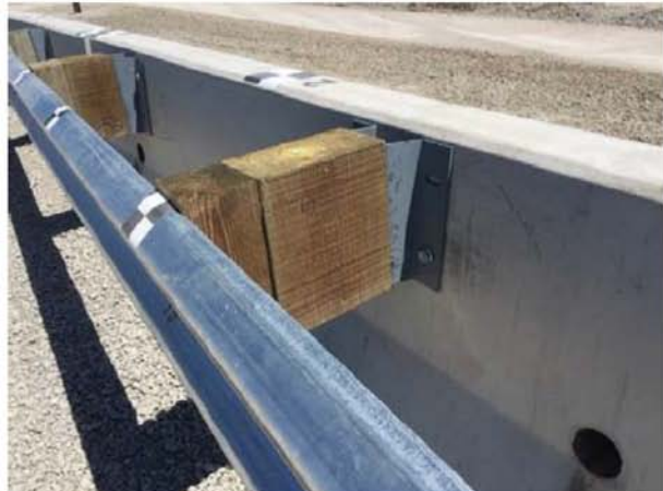
Figure 3. Guardrail-to-PCB transition system.
