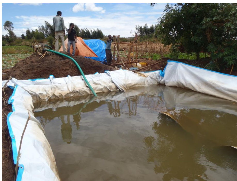
Figure 3. Pumping water out of temporary reservoir to irrigate a vegetable farm. Plastic membrane reduces seepage (3F Photo Archive).
