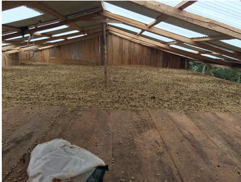
Figure 23. Rooftop drying area, Site 2c
