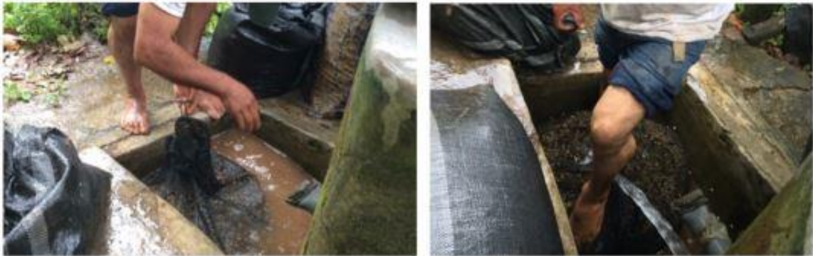
Figure 16. Modified use of cement washing tank, scrubbing in discharge channel
