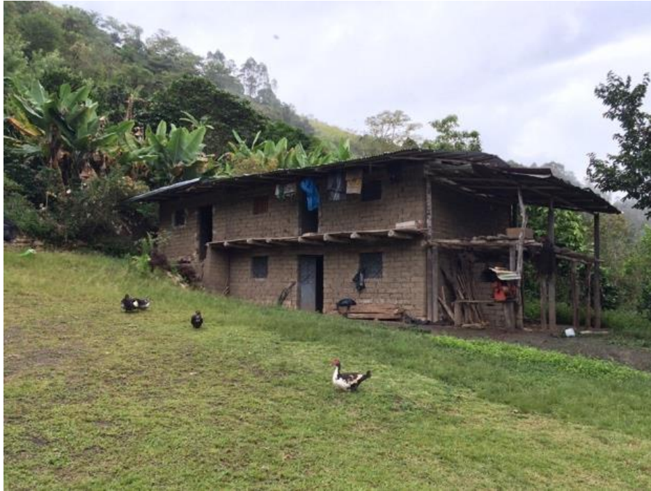
Figure 15. Field house for coffee storage, processing, and meals
