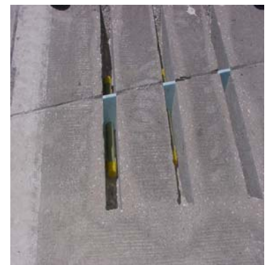
Picture 1.2: Placement of dowel bar chairs, dowel bars, and expansion joint.
