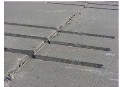
Picture 1.1: Removed pavement for new dowel bars.
