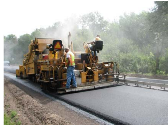
Picture 2.1: Application of topping on Louisville East section.
