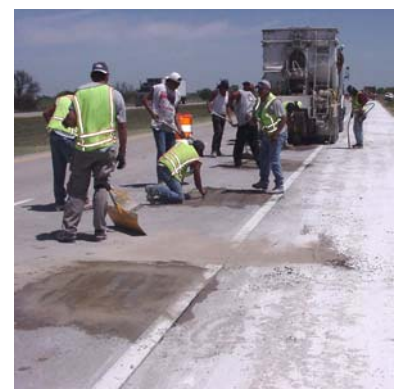
Picture 1.3: Placement of high strength grout.
