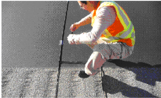
3. Installing tubes with a tape measure
