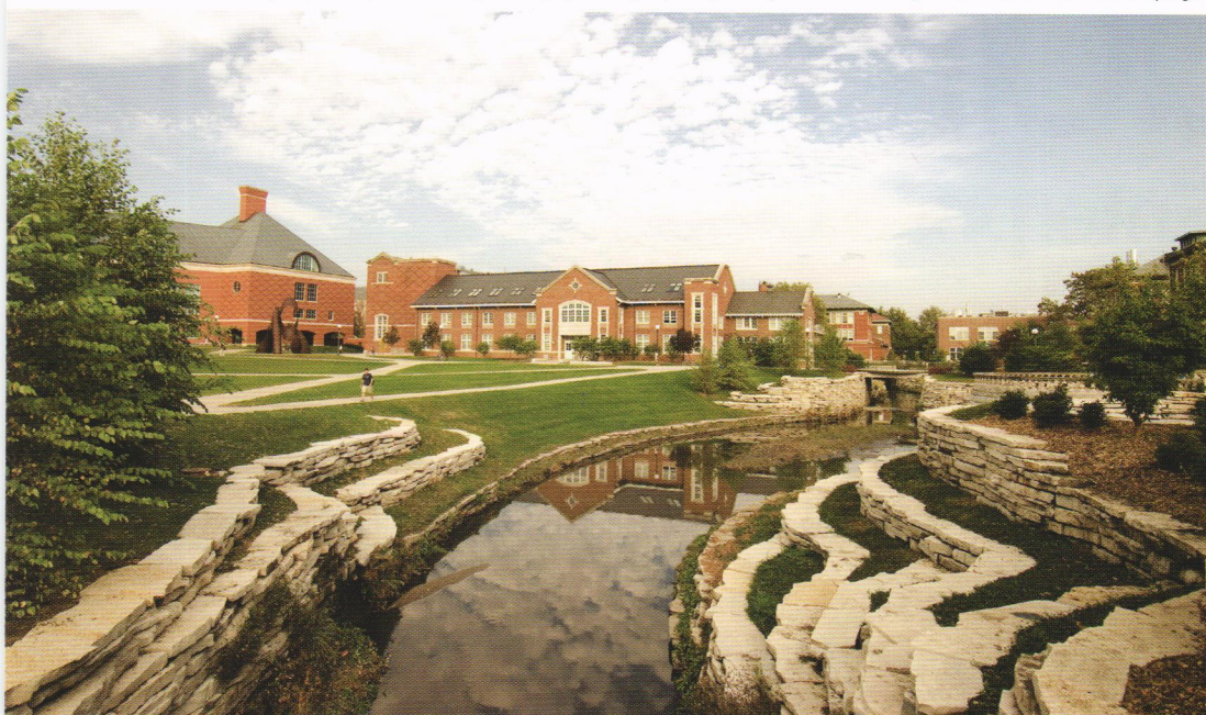
The Boneyard Creek (foreground) and the Engineering quadrangle (background) at the University of Illinois at Urbana-Champaign
