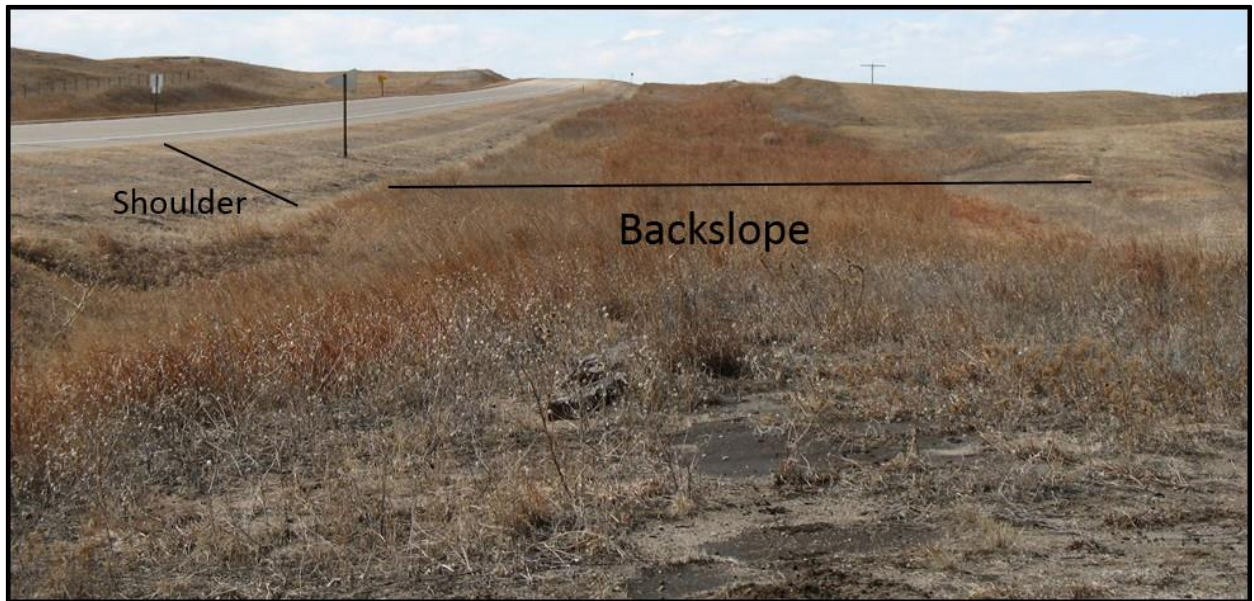
Figure 1. Example of shoulder and backslope locations along a roadside revegetation site. Near Nenzel, Cherry county, Nebraska. March 2008, credit: J. Soper.
