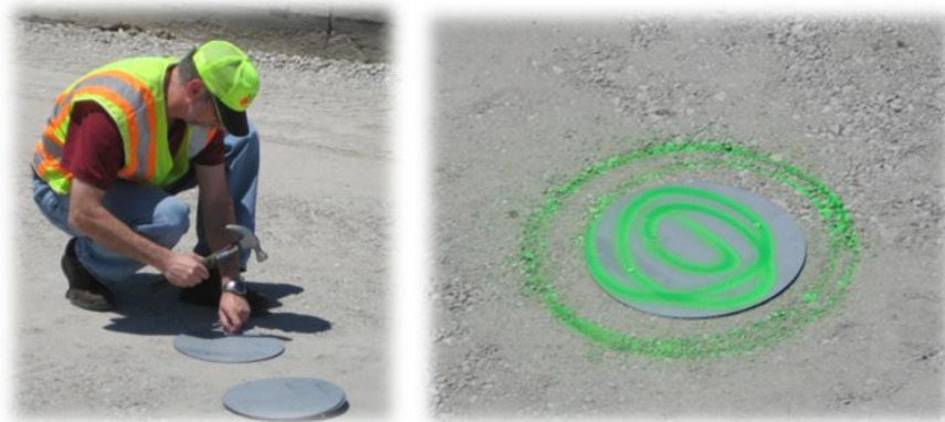
Figure 4.19 Placing reflector disks before paving Hwy 2.
