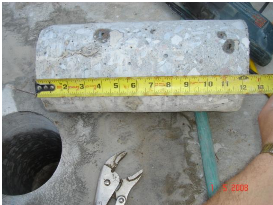
Figure 3.16 Thickness measurement using extracted cores
