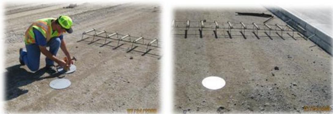
Figure 4.23 Placing reflector disk before paving I-80.
