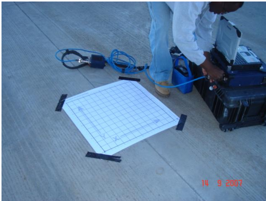
Figure 4.5 Grid setup at station 325 + 12
