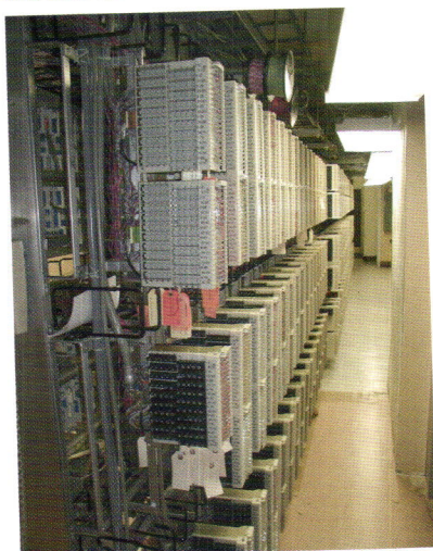
Figure 4. All cables end up at the main distribution frame (MDF). The MDF houses over 30,000 cable pairs from around the campus and is where the local exchange carrier (LEC) drops off trunks and network services to the university.
