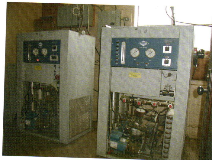
Figure 2. Air pumps Frankenstein and Godzilla pump air 24 x 7 through the LSU copper cable system.
