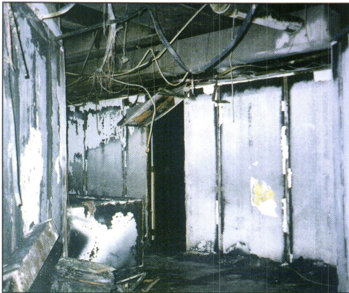
Fire damage results not only from combustion, but from water used in fire suppression and subsequent corrosion, from the greasy soot generated by certain plastics, and from chemical fallout.
