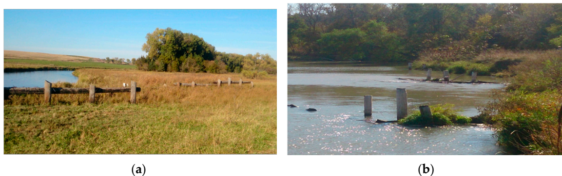
Figure 3. Jetties installed in 1950 at Site 5 (a) and in 2000 at Site 4 (b). Note the sediment that has accumulated over time in front of the jetties installed in 1950.
