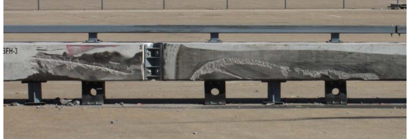
(c) System Damage
