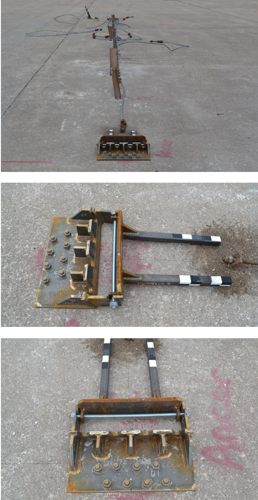
Figure 27. System Damage – Upstream Cable Anchor Bracket, Test No. HTCT-2
