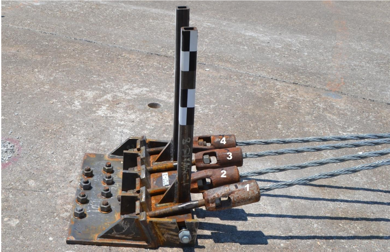
Figure 33. Cable Numbers at Upstream End Terminal, Test No. HTCT-3
