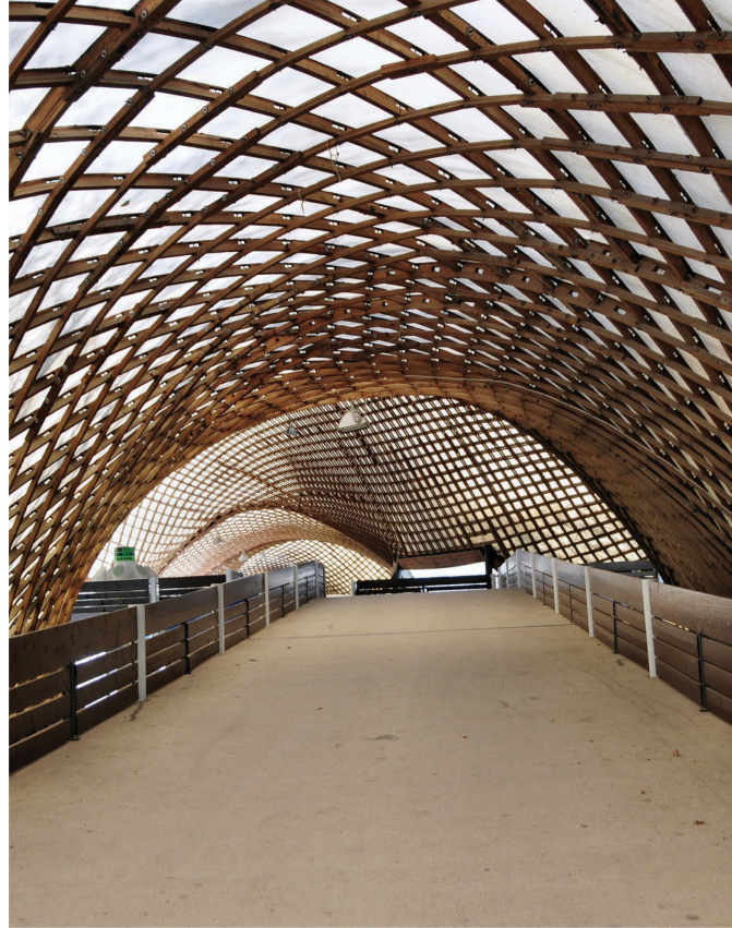
Figure 2.17 Timber shell roofs of the 1974 Mannheim Multihalle designed by Frei Otto (Linkwitz. 2014) Retrieved from: http://www.fastapp.com/index.php/en/projects-2/current/multihalle-in-mannheim
