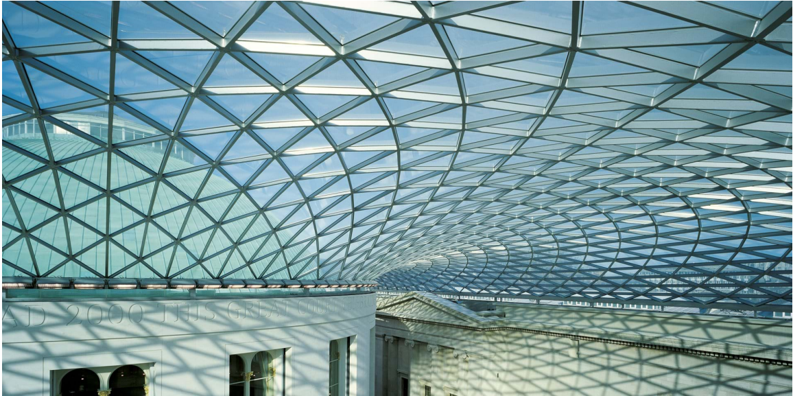
Figure 2.3 The British museum grid shell designed by Norman Foster. Retrieved from: https://www.fosterandpartners.com/projects/great-court-at-the-british-museum/
