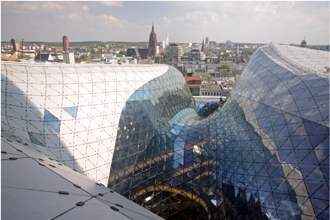
Figure 2.4 Myzeil's facade in Frankfurt was designed by alternating panels of glass and steel by Massimiliano Fuksas. Retrieved from: https://www.archdaily.com/243128/myzeil-shopping-mall-studio-fuksas
