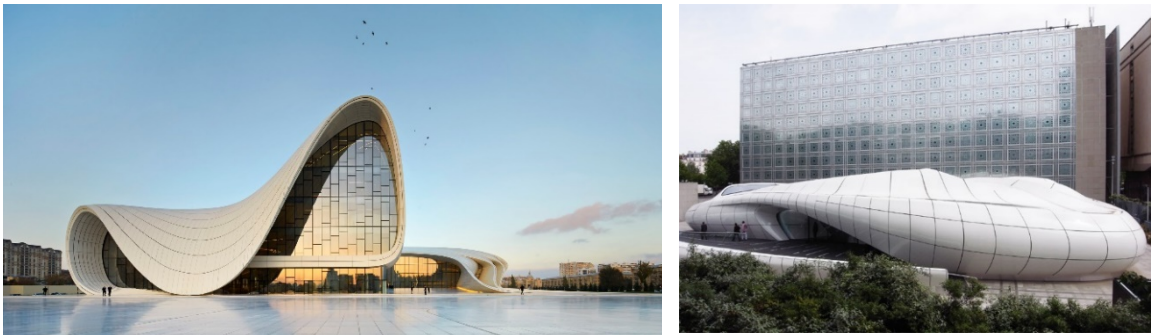
Figure 2.5 The tessellated skin of Heydar Aliyev Center (left); and Chanel Mobile Art Pavilion (right) designed by Zaha Hadid Architects. Retrieved from: http://www.zaha-hadid.com/architecture/heydar-aliyev-centre/
